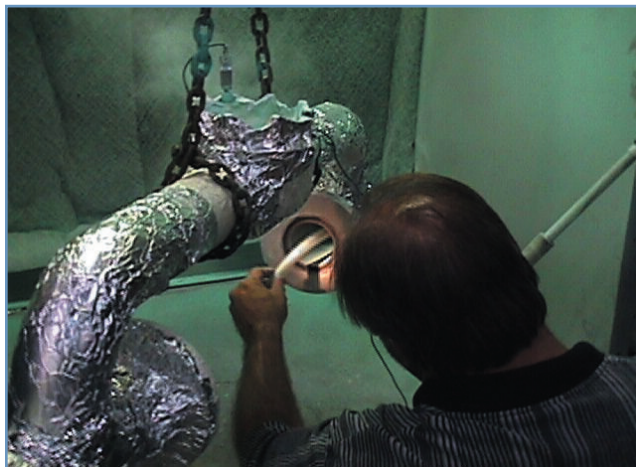
Figure 6. Coating of piping Segment 2 assembly with flexible extension.
