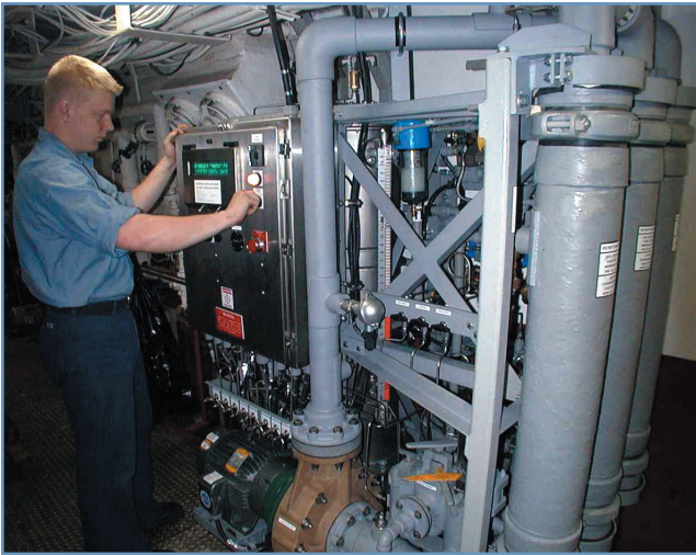
Figure 4. Engineering development model 10 gpm oily waste membrane system.
