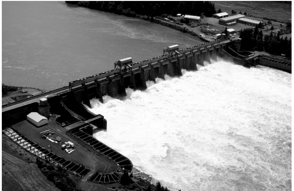
Figure 5: Water Being Released at Bonneville Dam
