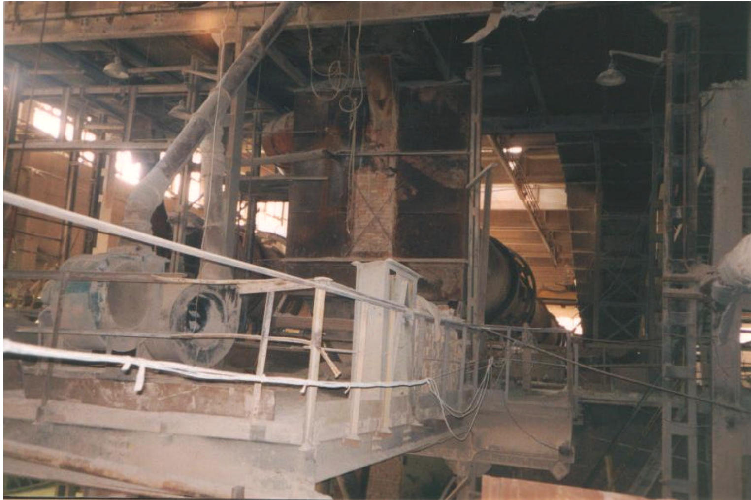
1993. Interior of pipe shop of abandoned ceramics factory. Large, third-story windows on left face northwest.
