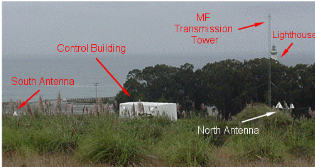
Figure 67 USCG Pigeon Point DGPS Reference Station
