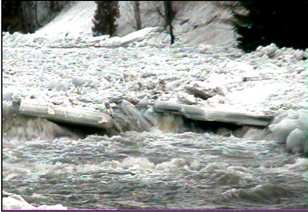
Figure 2. Ice jammed on the Lamoille River at the Hardwick, Vermont, ice control structure during ice cover breakup on 28 February 2000.
