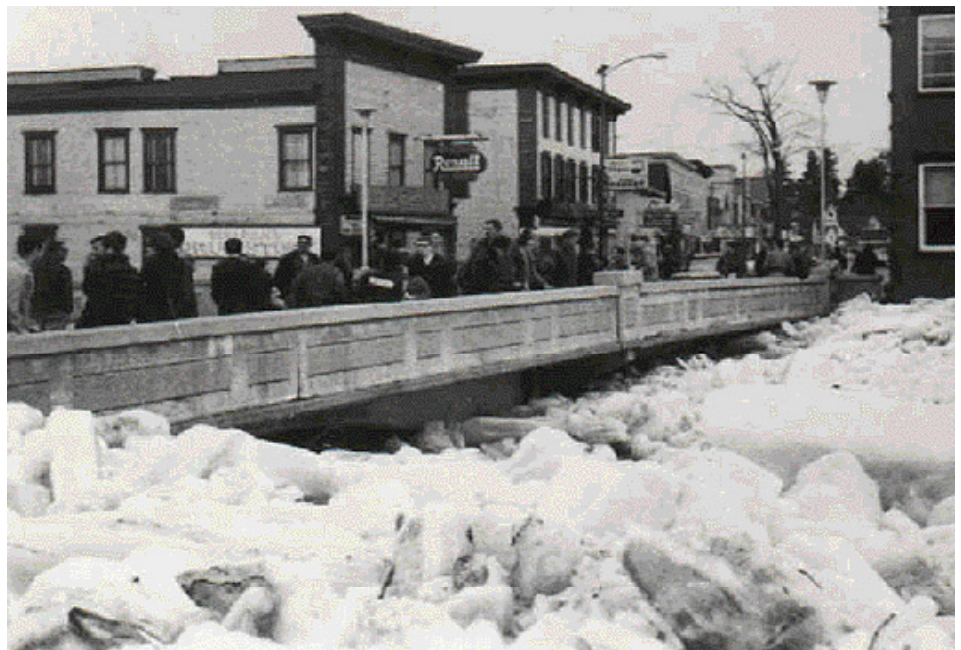
Figure 1. March 1968 ice jam on the Israel River at Lancaster, New Hampshire. Ice jams increased in frequency and duration here following the failure or removal of four dams on the river between 1936 and 1950.
