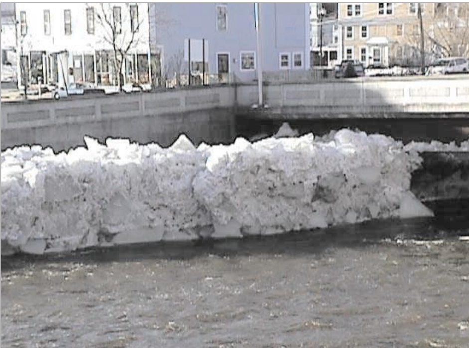
Figure 1. Shear wall left behind following failure of the January 1999 ice jam on the Israel River in Lancaster, New Hampshire. Note ice on low steel of bridge. (Photograph courtesy of www.greatnorthwoods.org .)
