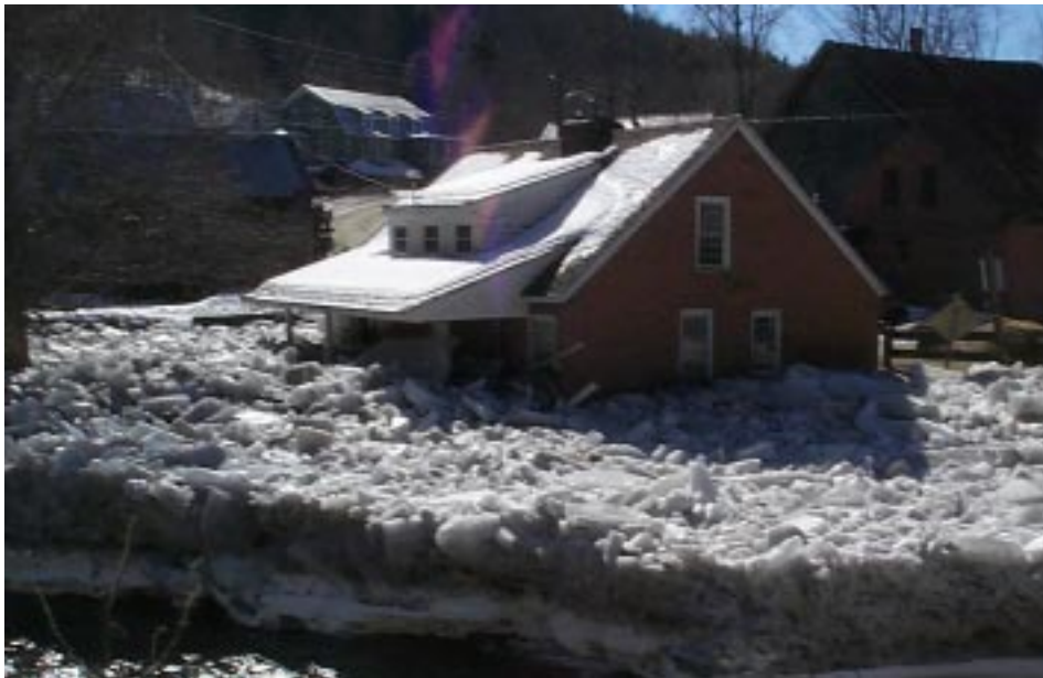
Figure 1. Surrounding areas were flooded when ice destroyed the Tunbridge Mill covered bridge in March 1999.
