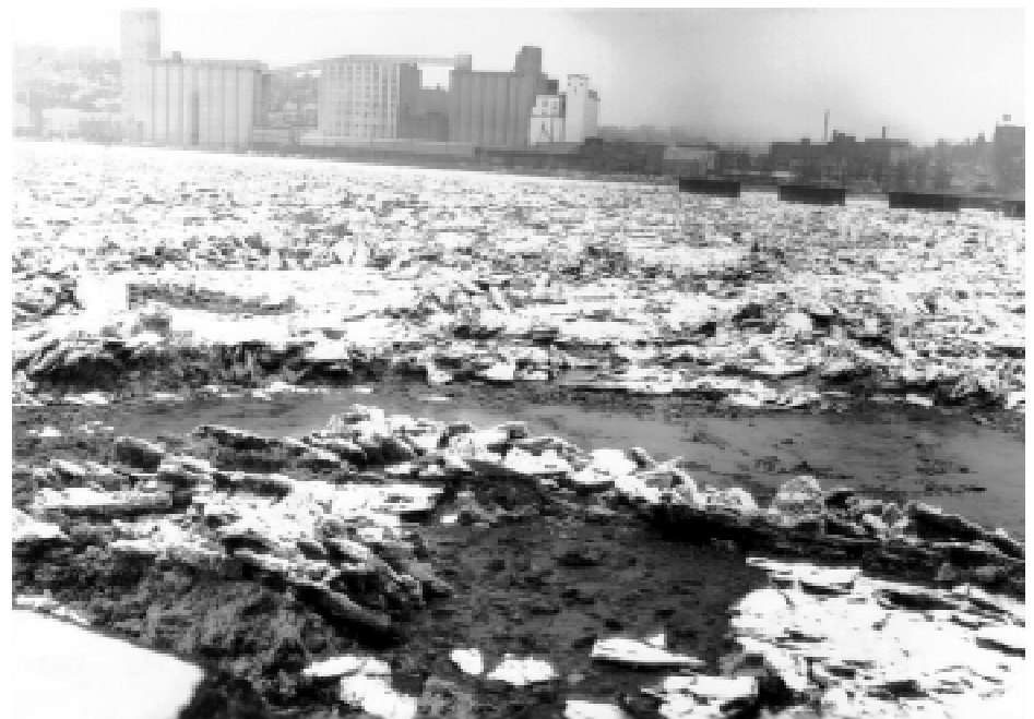
Figure 1. View from Lock and Dam 26 toward Alton, Illinois, showing ice jammed upstream from the dam (29 January 1960).
