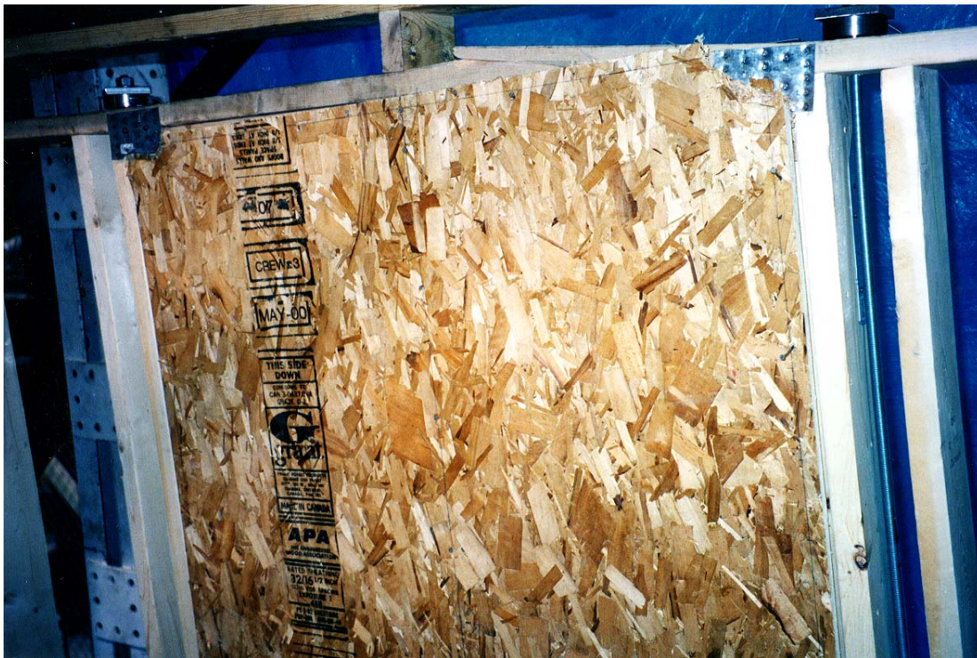
Figure 40. Top plate splitting above the right side of the OSB.
