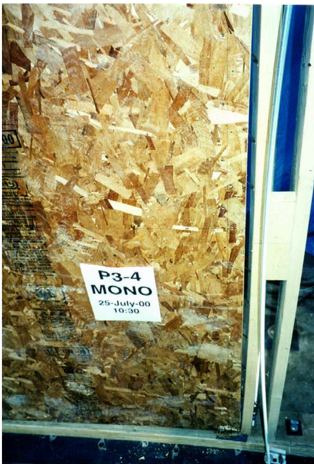
Figure 49. Inset panel detached from 2x6 frame.
