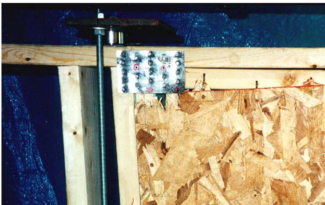
Figure 36. Block shear pullout of OSB from TP35 nailing plate.
