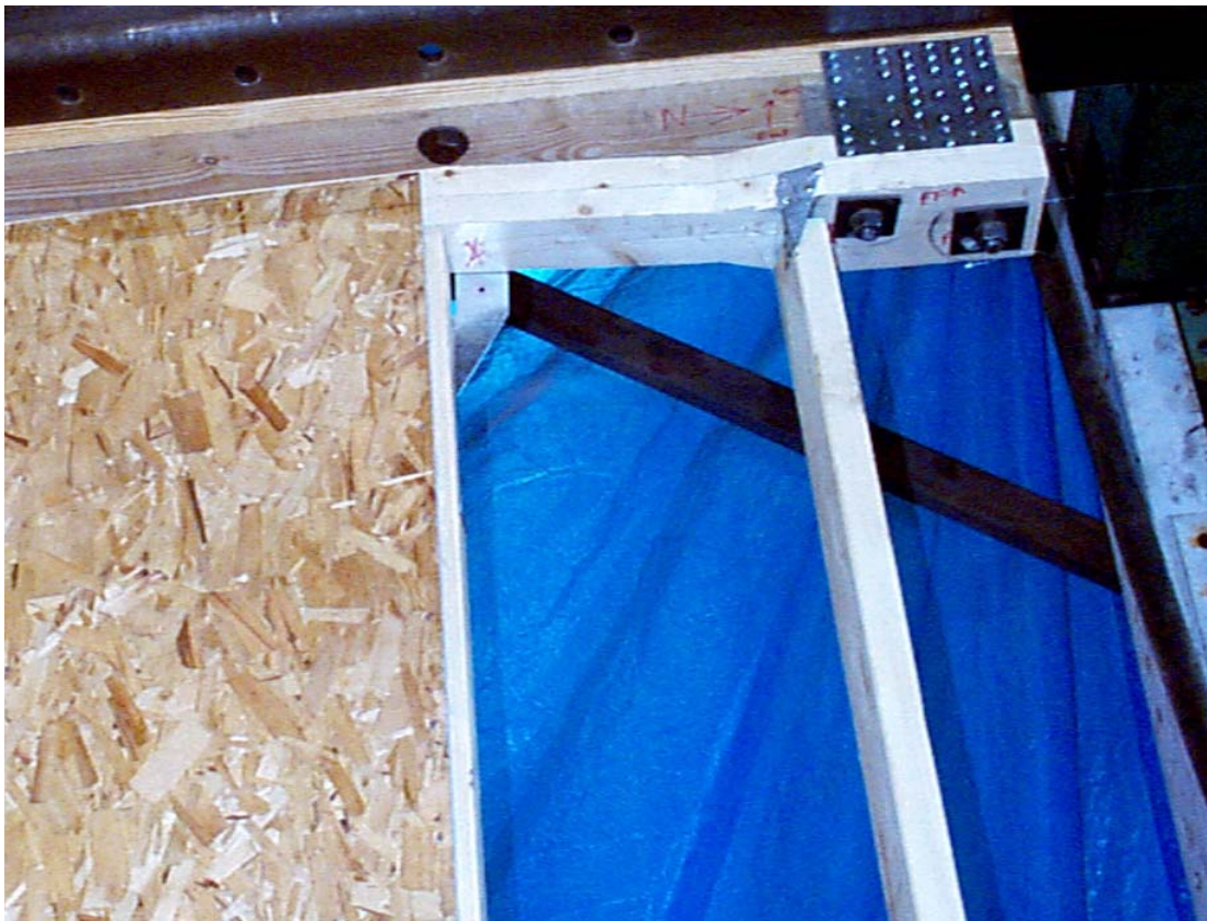
Figure 73. Bending failure (cracking) of the top plate above the right edge stud.
