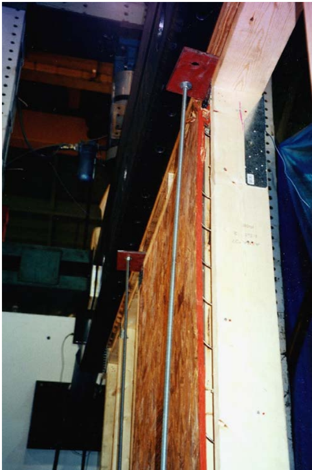
Figure 44. OSB outside the 2x6 frame and nail pullout along right vertical edge of panel.
