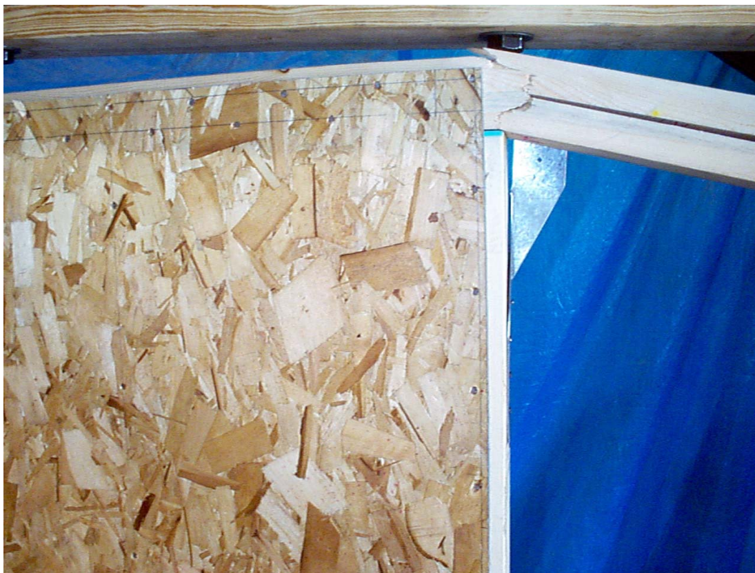
Figure 76. Bending failure of the 2x4 top plate on P3-6 CUREE2 panel.
