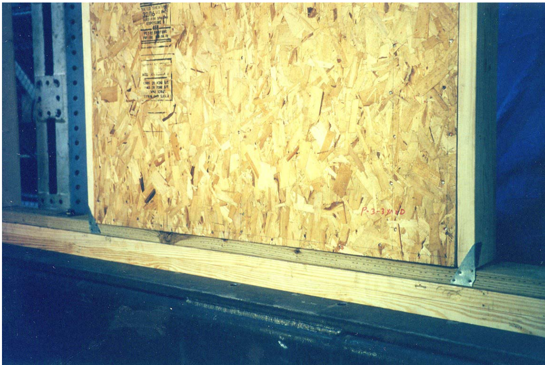
Figure 60. Nail yielding and OSB crushing in P3-3M CUREE1 test.
