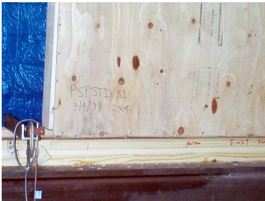
Figure 82. Bottom left corner of the PSP-Std-SPD1 panel showing plywood to bottom plate nail connection failure and stud lifting.
