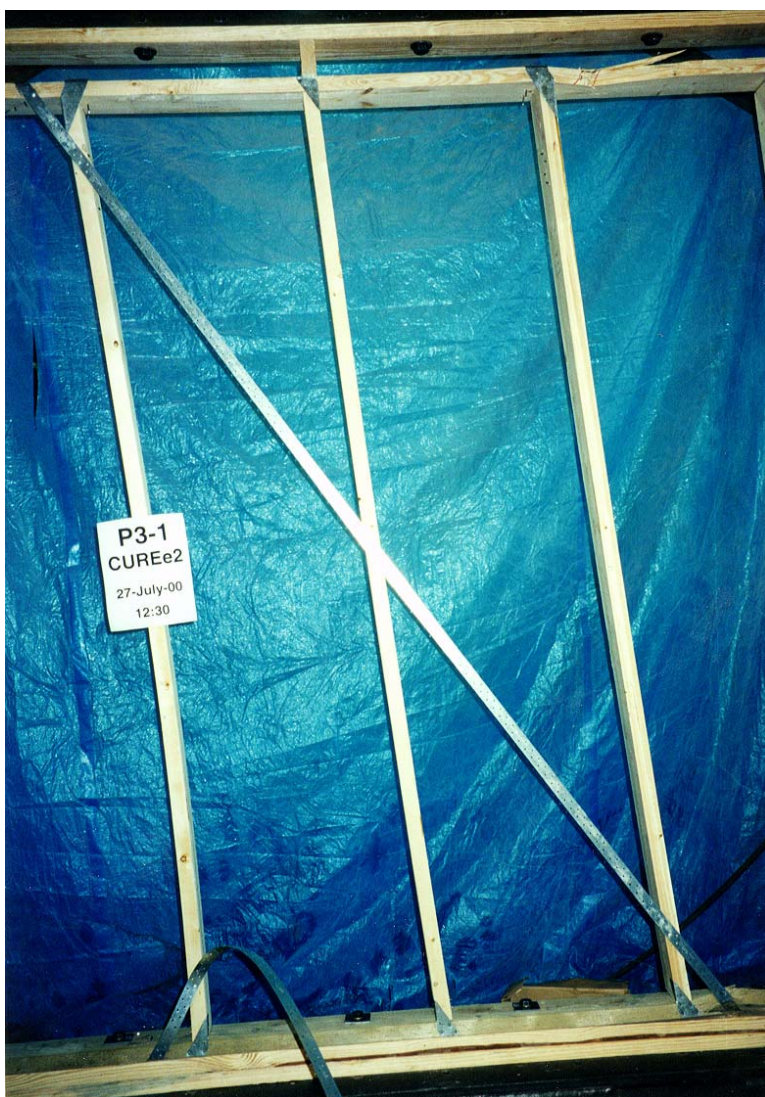
Figure 31. Damage state after completion of P3-1 CUREE2 test (7-7).
