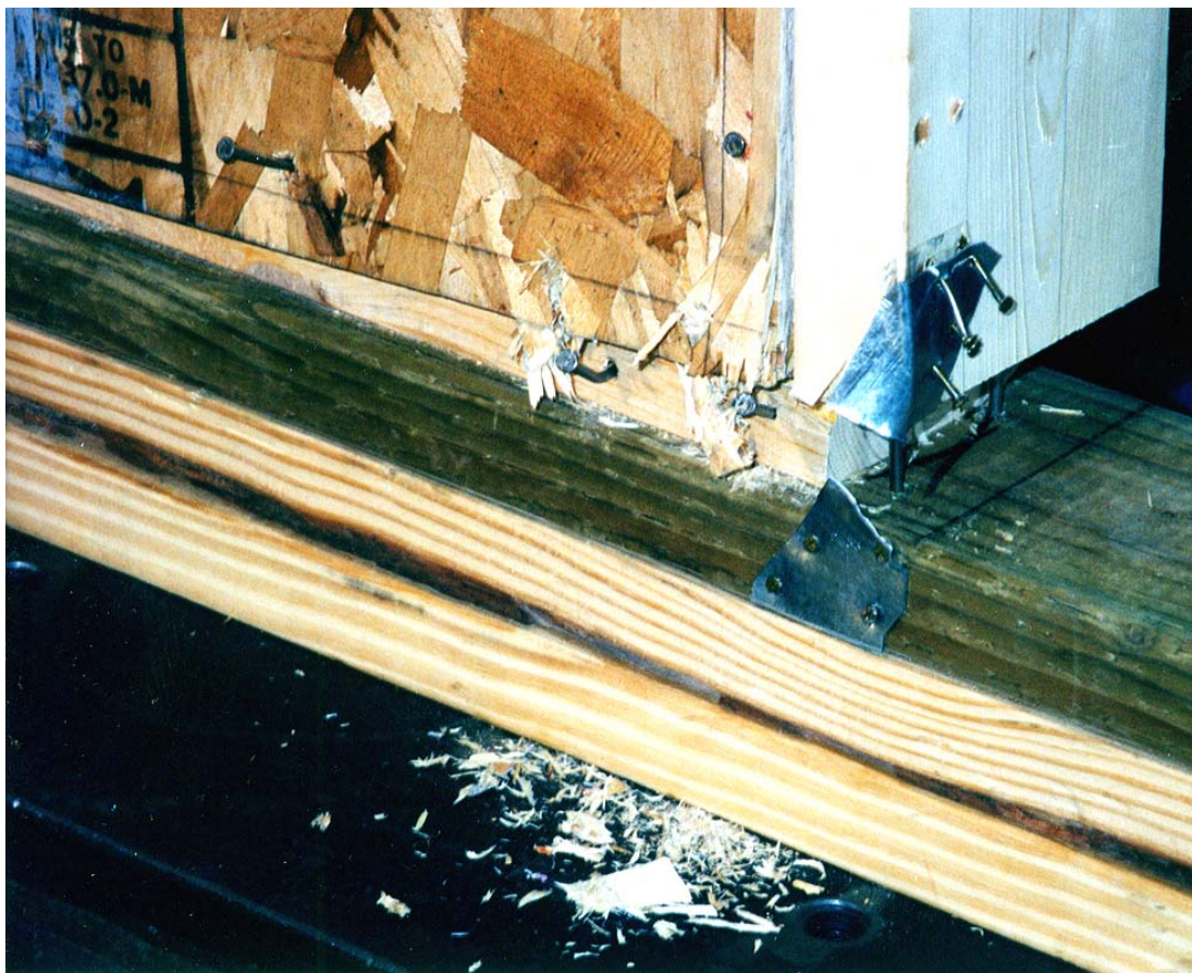
Figure 80. Failure of H4 ties, OSB, bottom plate, and nail connections of P3-7 CUREE2 panel.
