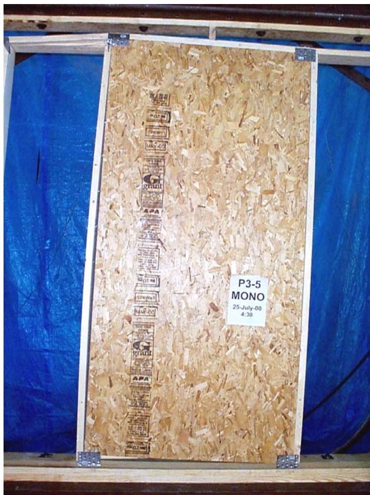
Figure 51. Top plate bending and nail yielding along OSB left edge.
