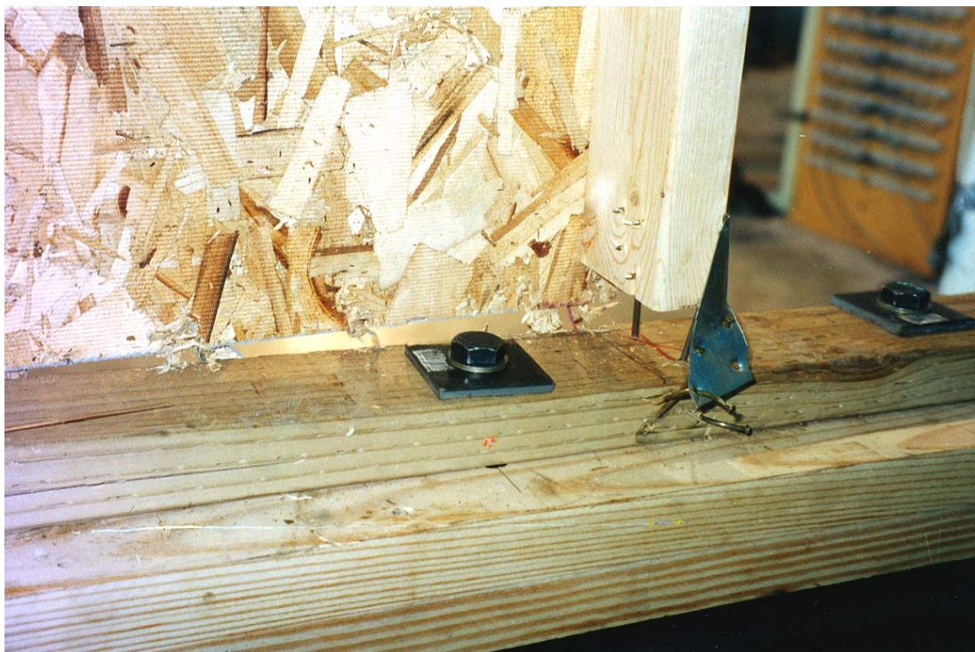
Figure 75. Interior face of P3-6 CUREE2 panel showing OSB nail and H4 tie nail failure.
