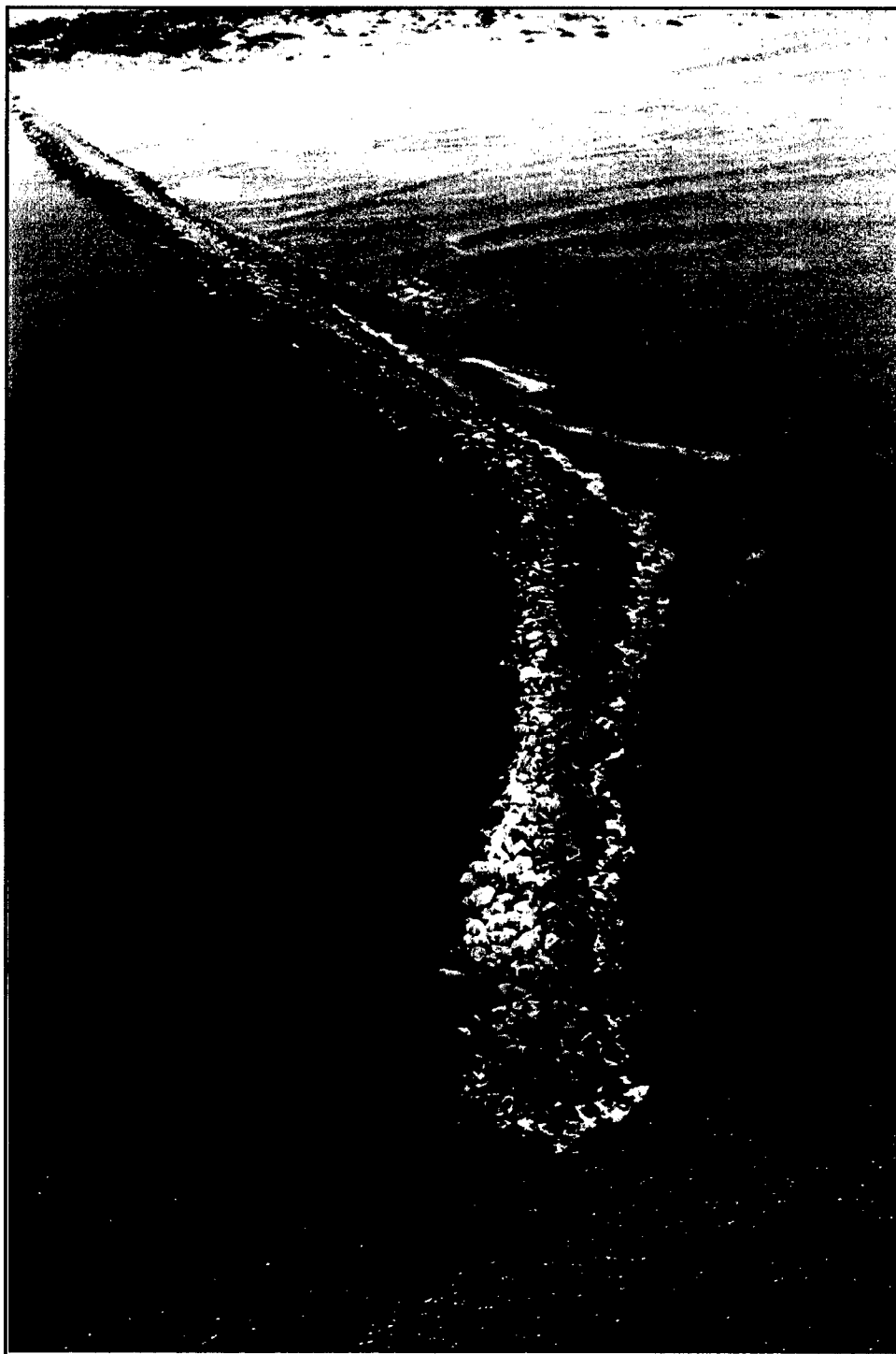
Figure 7. Aerial view of south breakwater
