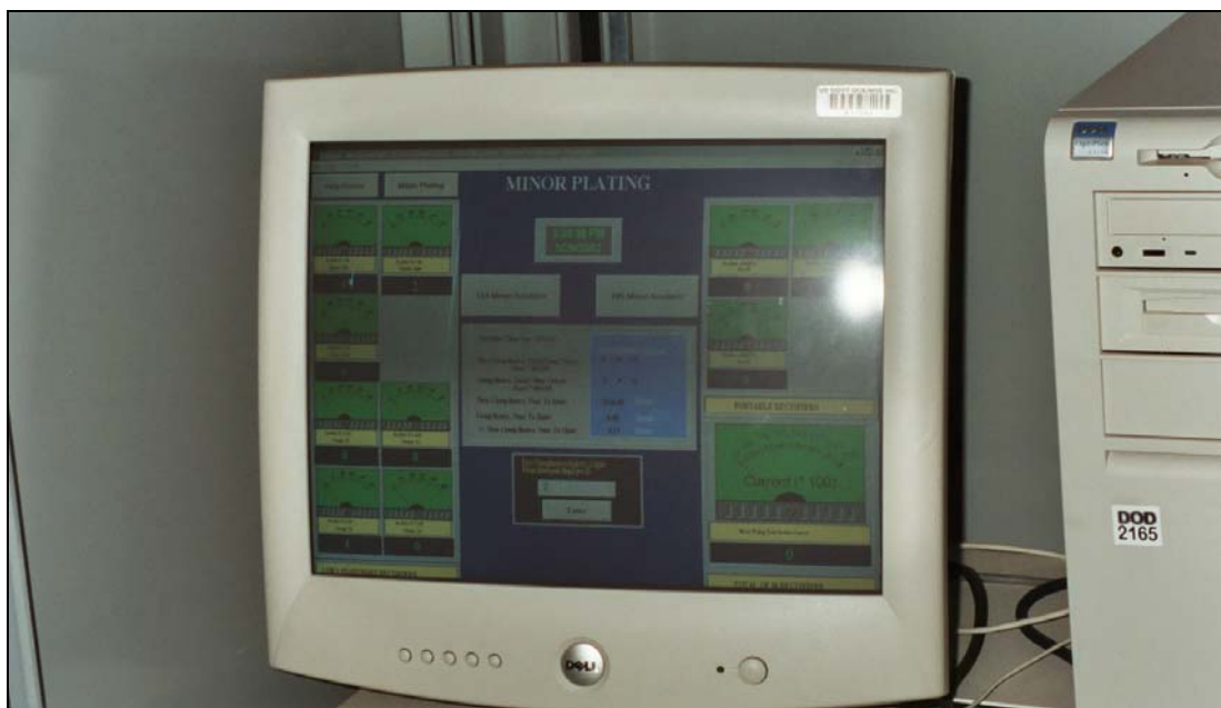
Figure 8. Chrome plating scrubber air monitoring NESHAP compliance computer.
