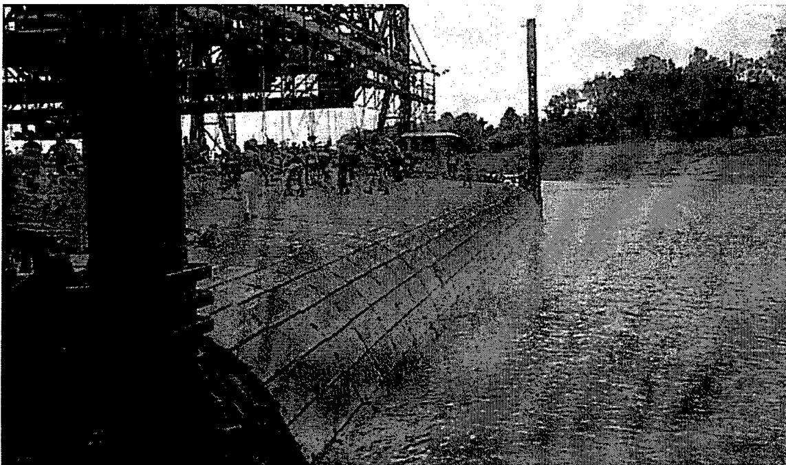
Figure 22. Machinery for laying articulated mattresses on riverbanks
