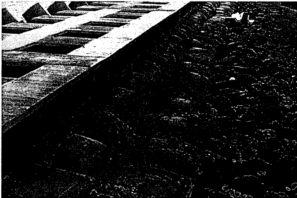
Figure 8. 2,270-kg (2.5-ton) high-strength concrete units used on harbor side of structure
