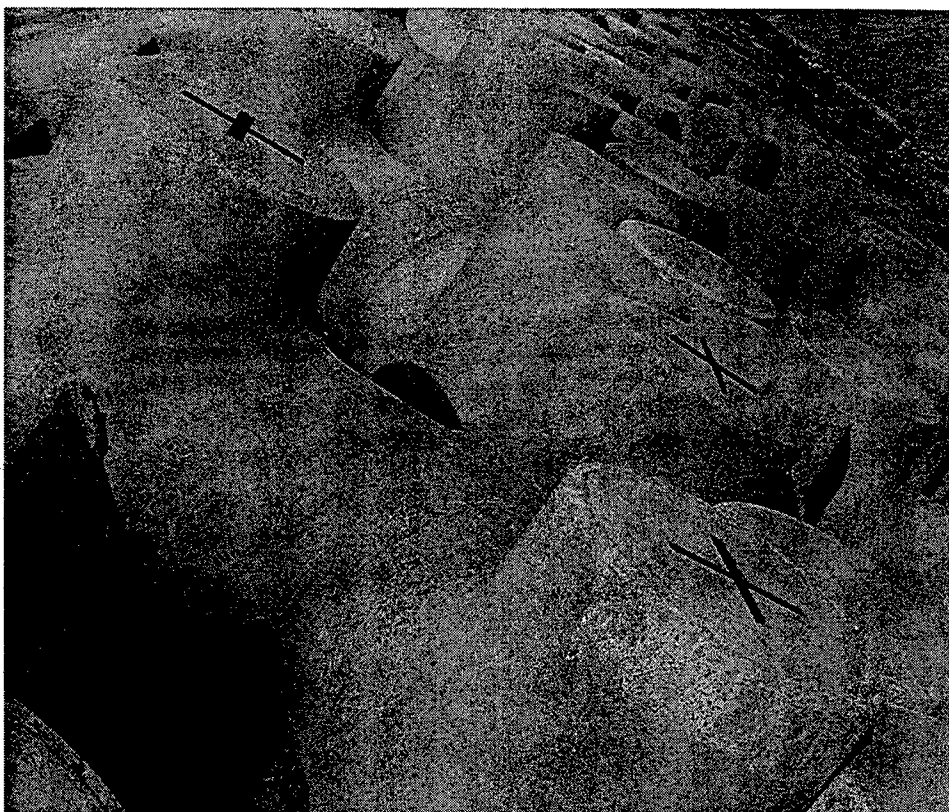
Figure 16. View of a targeted tribar (three targets established)
