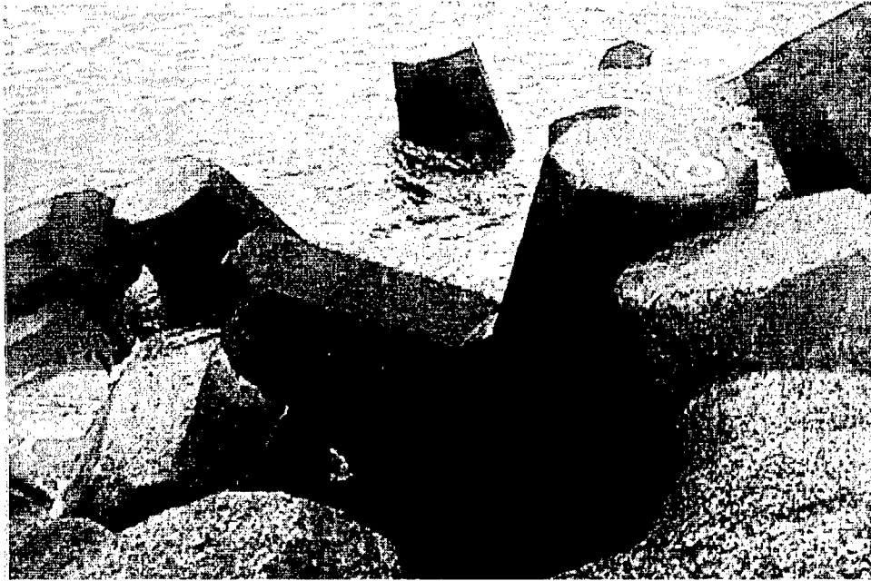
Figure 30. Dolos with shank-fluke break
