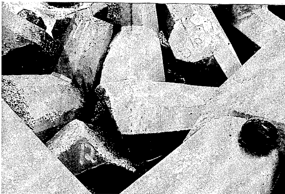
Figure 29. Dolos with fluke-shank break
