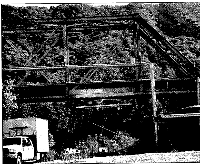
Figure 2. Railroad bridge at HAAP, TN, with overcoated test areas.
