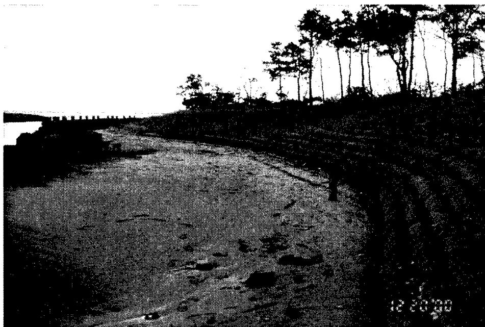
Fig. 8: Well designed bioengineering for coastal bank erosion control
