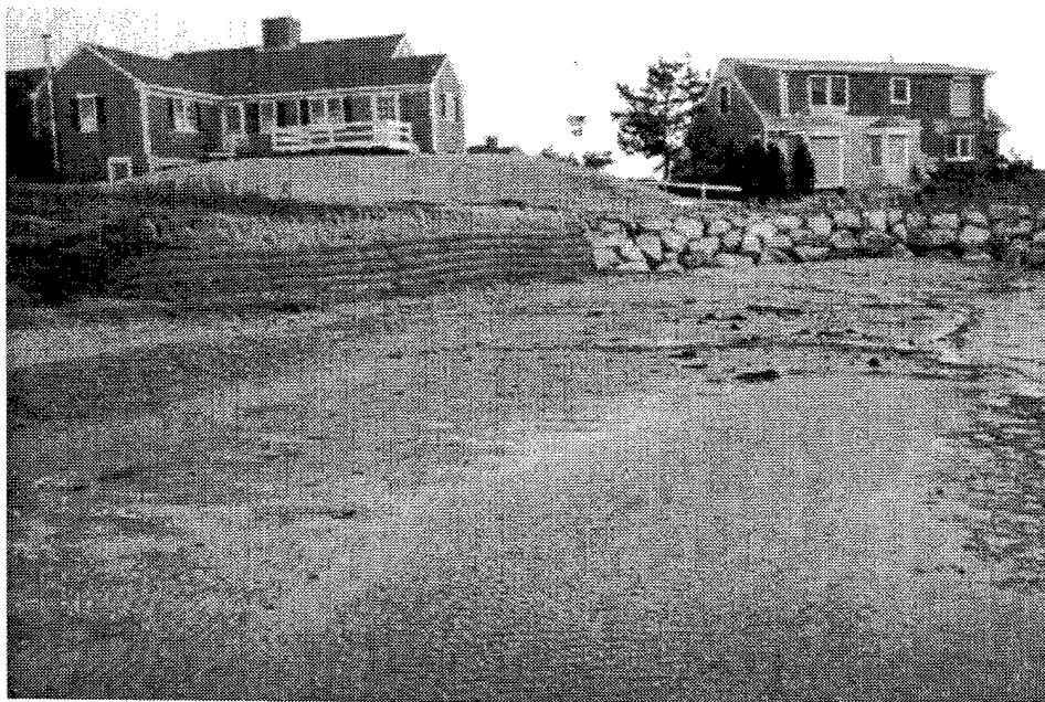
Fig 36. Using fiber rolls to construct a return
