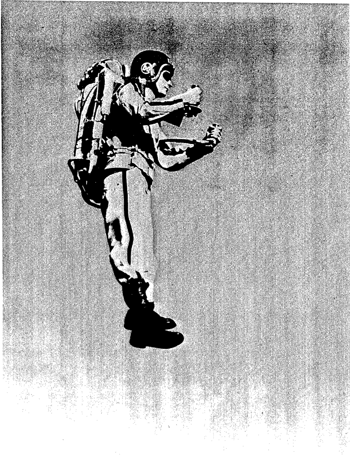
Figure 3. Bell Rocket Belt, Predecessor to the Bell Jet Belt
