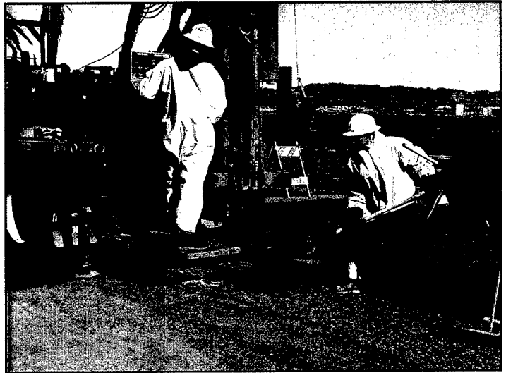
Hollow-stemmed auger being used at 5th Street on Treasure Island, January 2001
