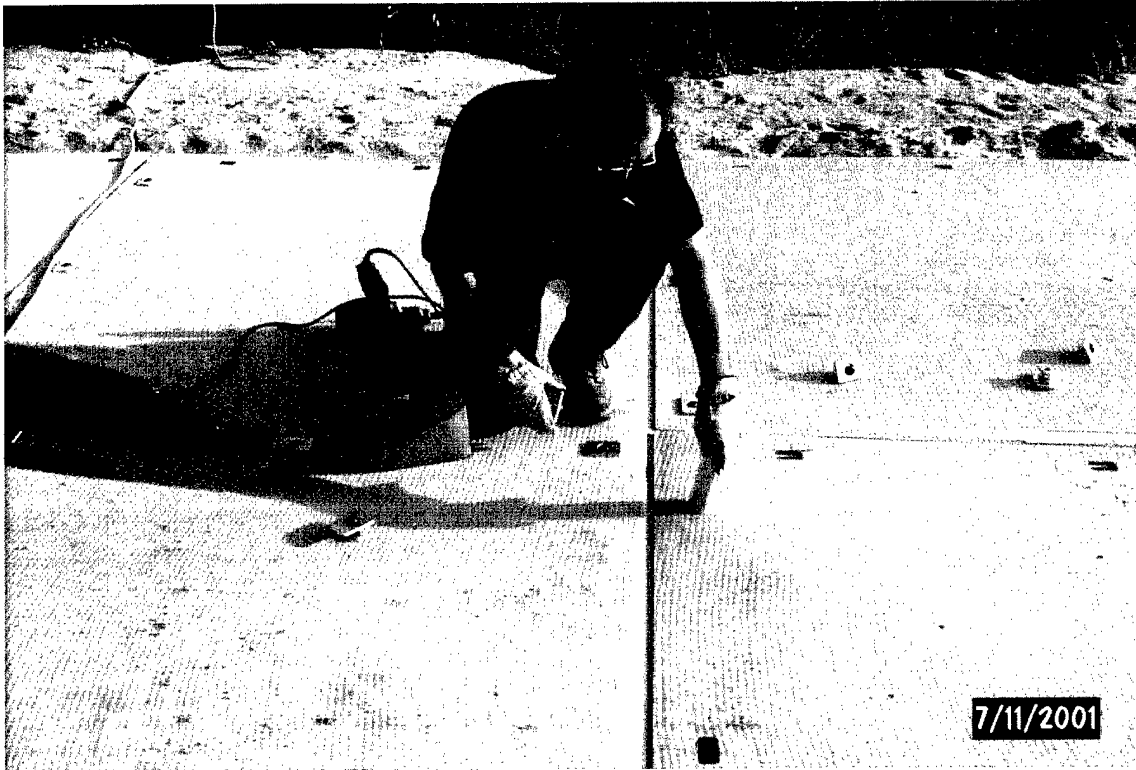
Photo 41. Aligning mat panel holes using alignment tool
