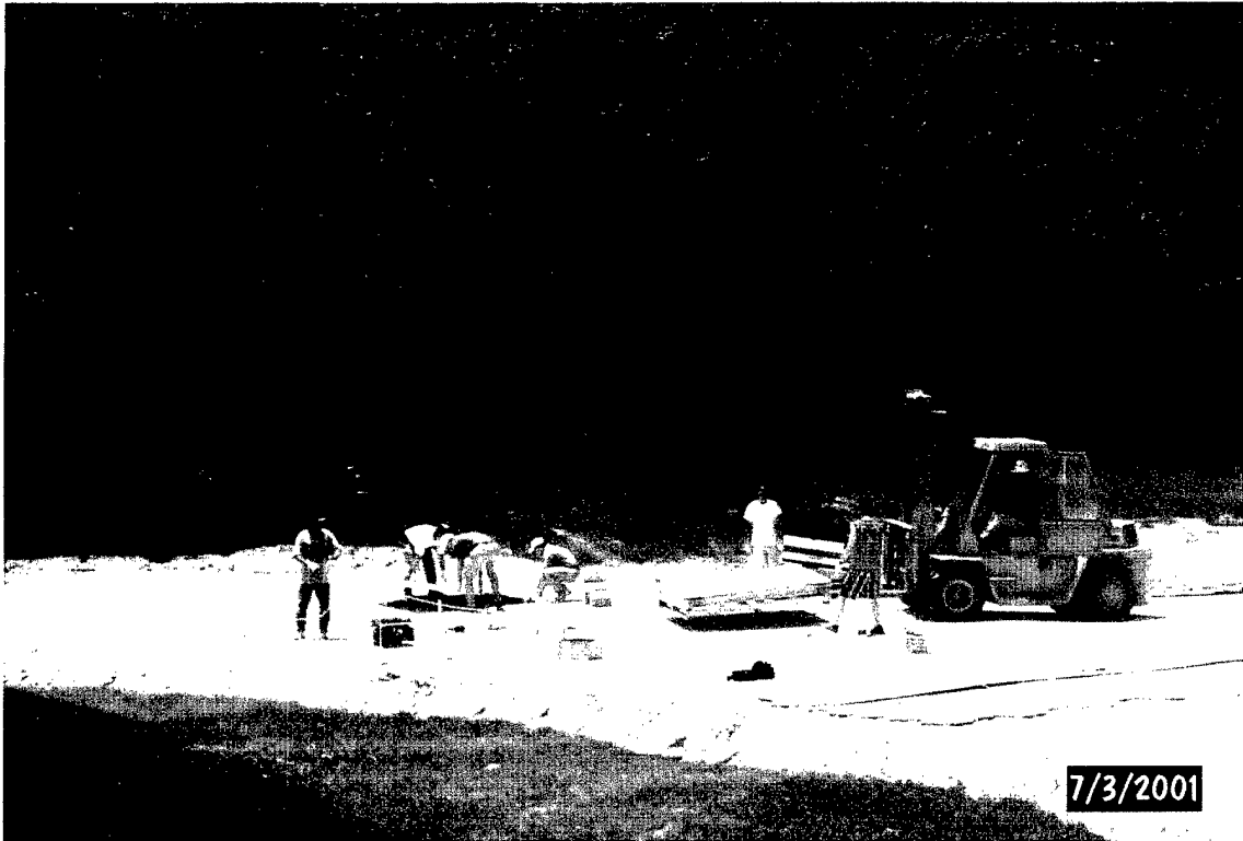
Photo 37. Forklift delivering MP mats to installation site
