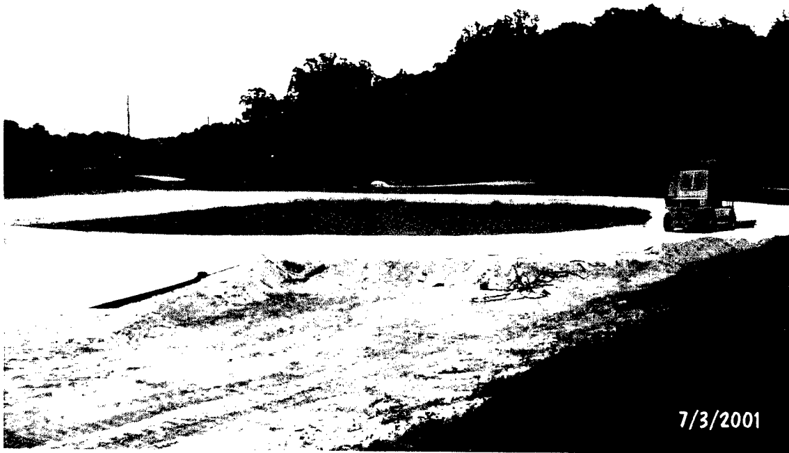
Photo 27. Item 1 50-ft radius curve section
