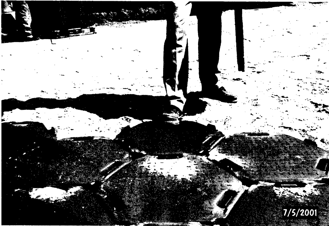
Photo 55. Allround hexagonal plastic mat installation – Step 3
