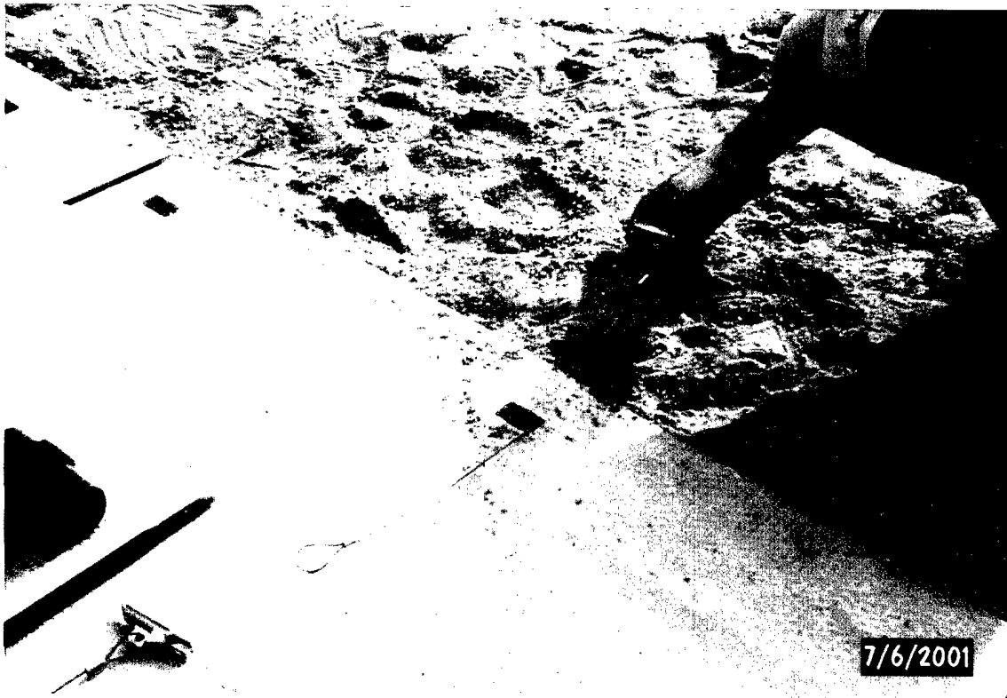
Photo 47. Anchor cable inserted throughout the mat hole
