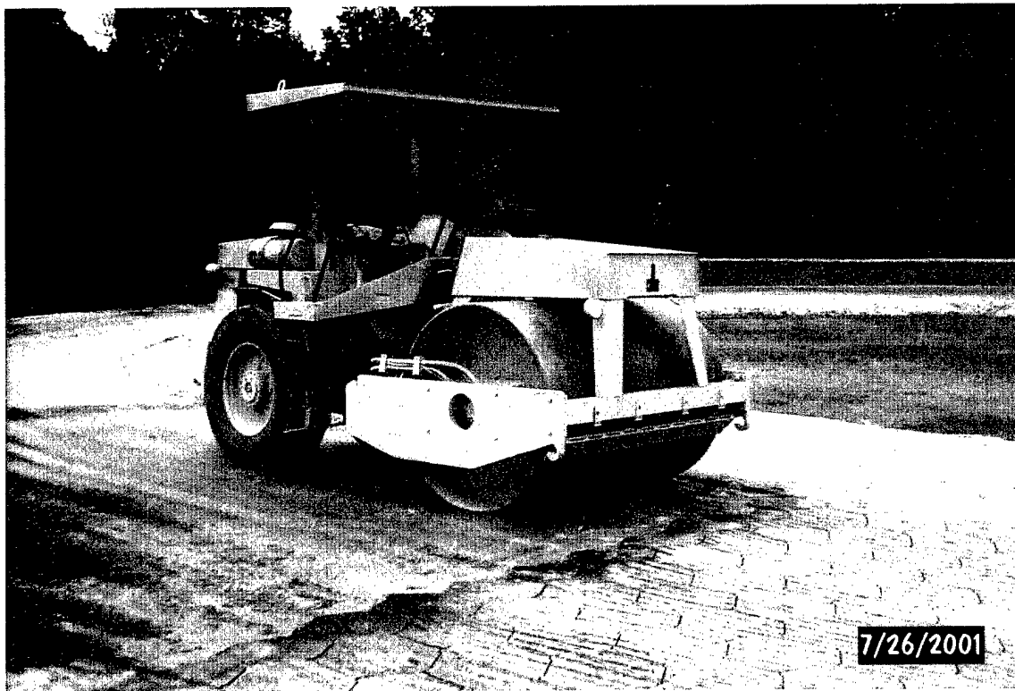
Photo 34. Special hexagonal plastic mat and 75-ft radius curve sand-geofiber section transition zone
