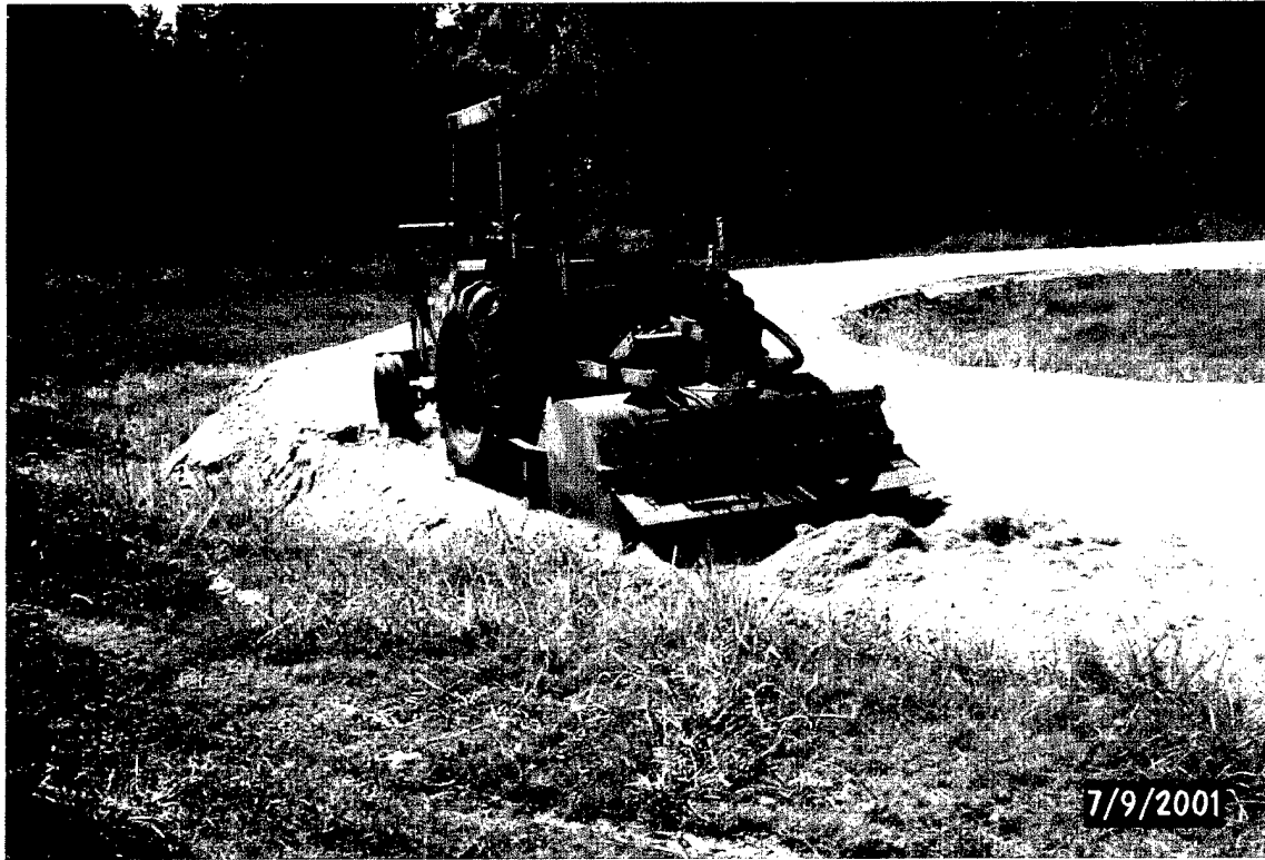
Photo 69. Mixing geofibers into the sand with self-propelled rotary mixer
