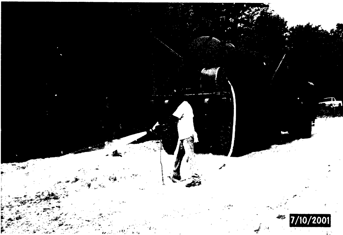
Photo 72. Watering sand-geofiber item prior compaction
