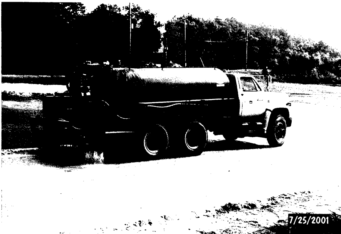
Photo 76. Spraying Road Oyl over the sand-geofiber
