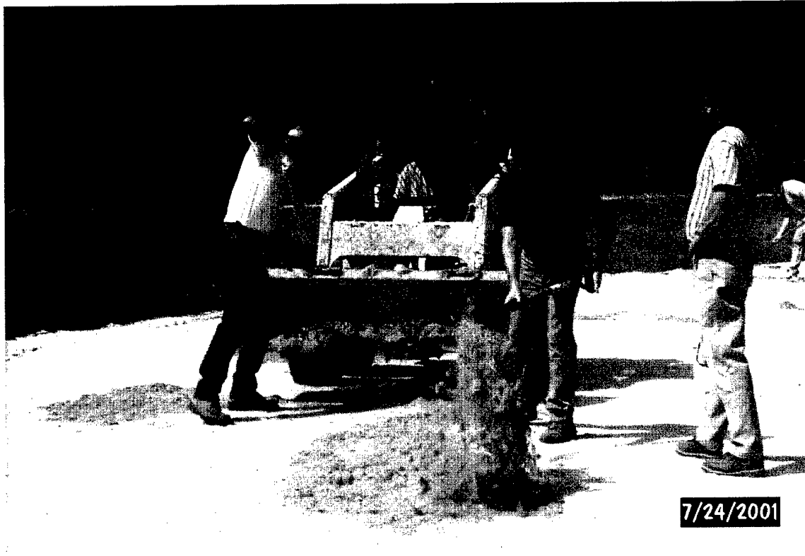
Photo 77. Patching with sand-geofibers
