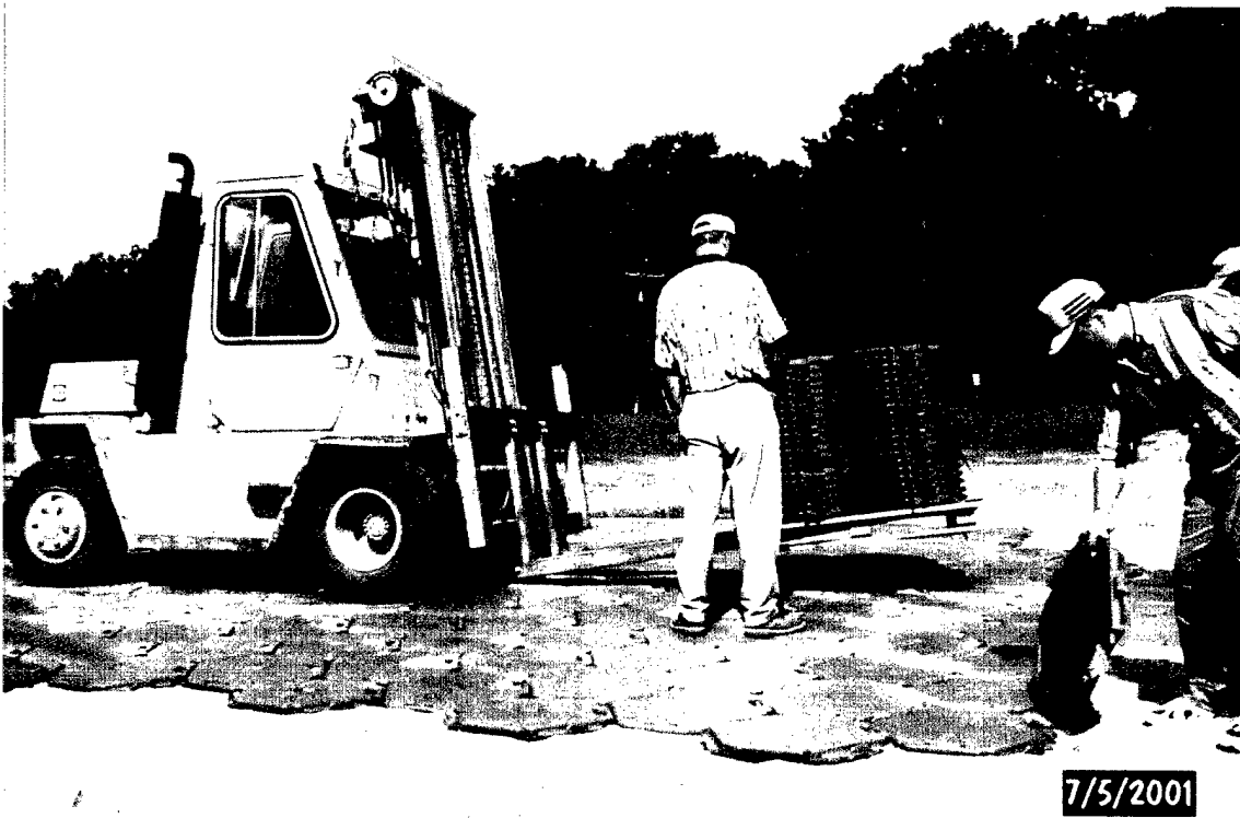
Photo 52. Forklift delivering Allround hexagonal mats to installation site
