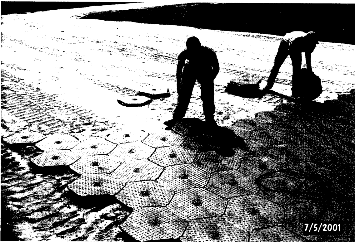
Photo 60. Special hexagonal plastic mat – Step 2 and 3
