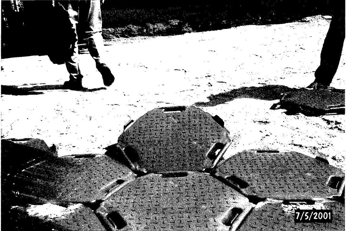
Photo 54. Allround hexagonal mats installation - Step 2
