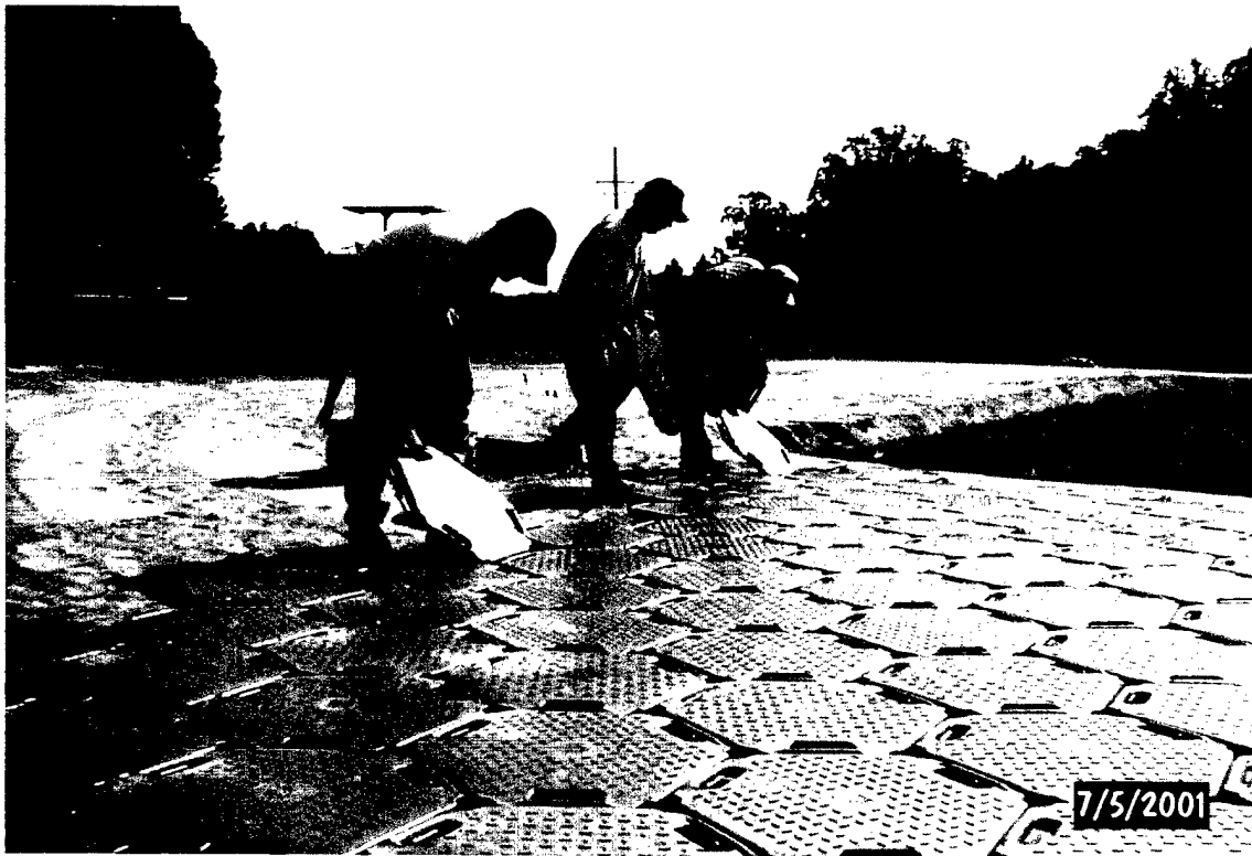
Photo 56. Allround hexagonal mats installation progress
