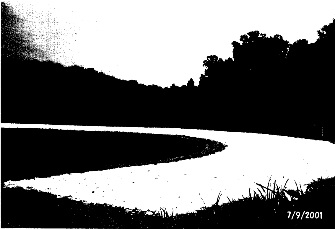
Photo 68. Item 3 after spreading the geofiber and prior mixing
