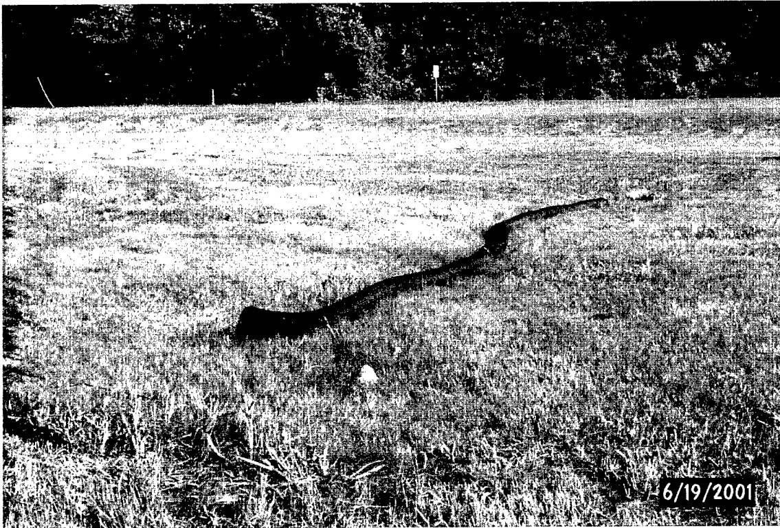
Photo 18. Placement of the drainage pipe
