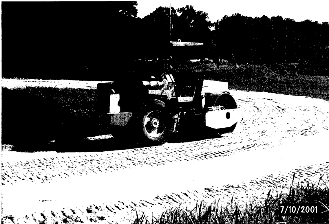
Photo 73. Compaction of the sand-geofiber item
