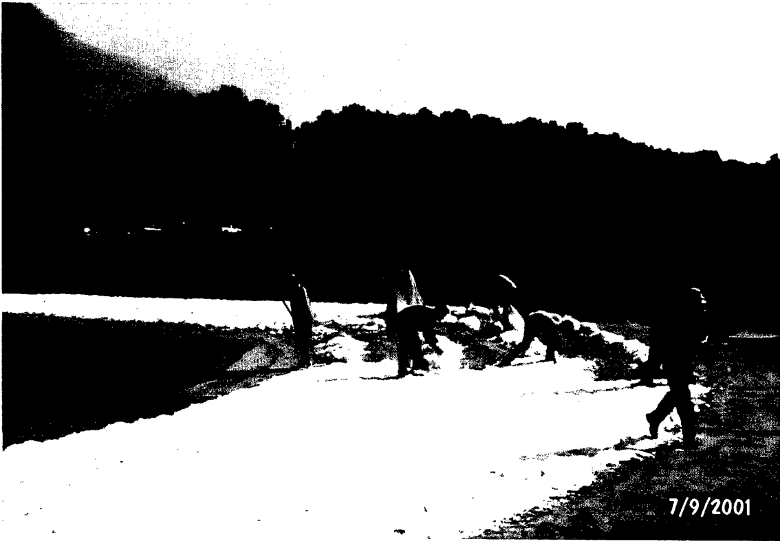
Photo 67. Spreading geofibers over the sand layer
