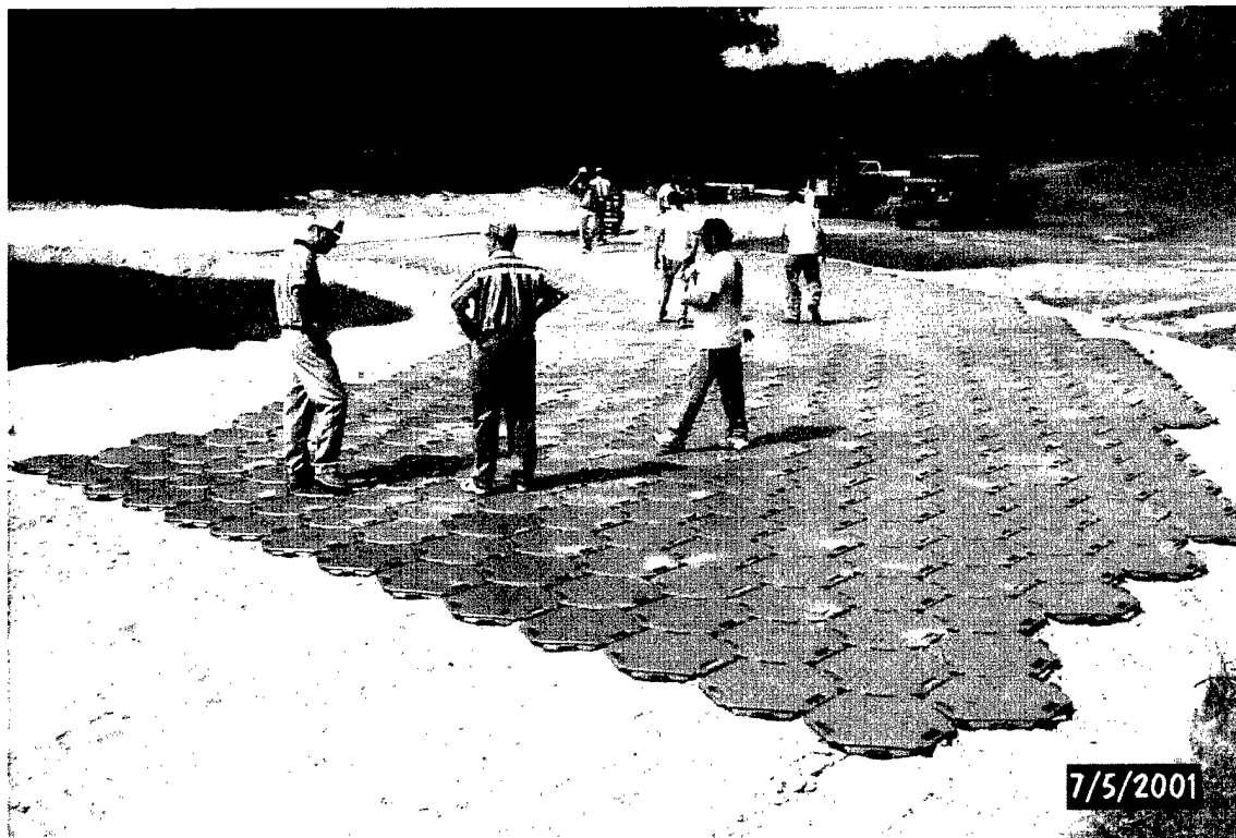
Photo 58. Completion of Allround hexagonal mat section
