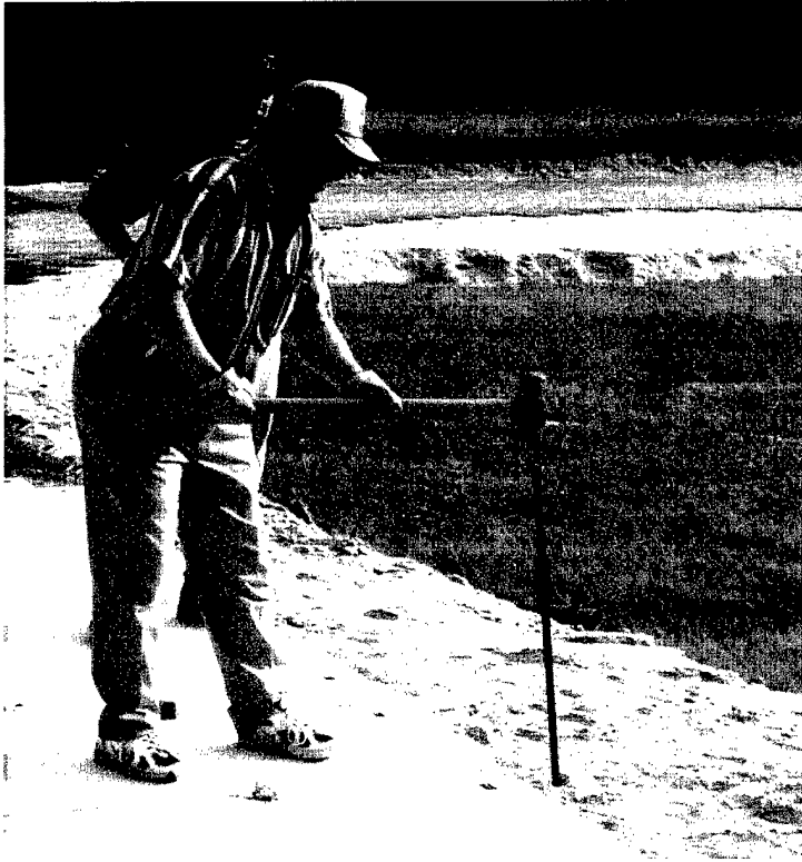
Photo 49. Driving the anchor using the steel driver rod
