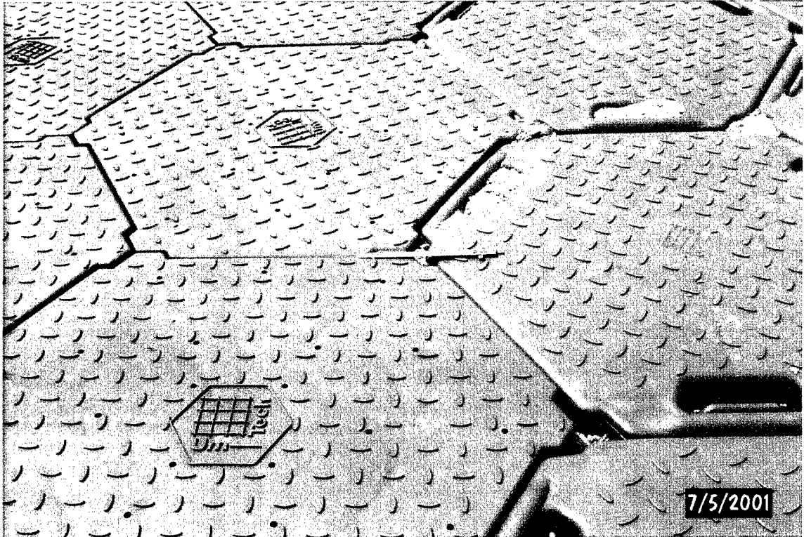
Photo 62. Hexagonal plastic mats transition zone close-up
