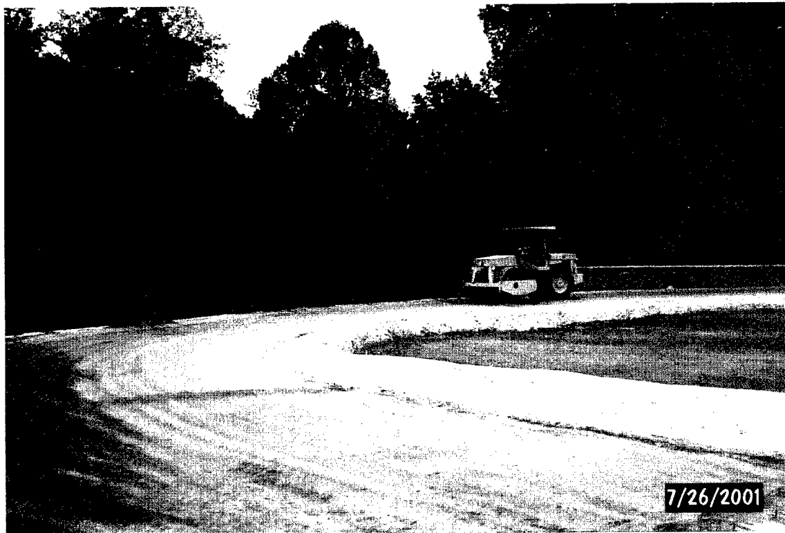
Photo 78. Compaction to seal the sand-geofiber surface
