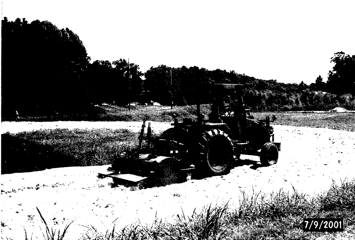
Photo 70. Sand-geofiber item after 4 passes of the rotary mixer
