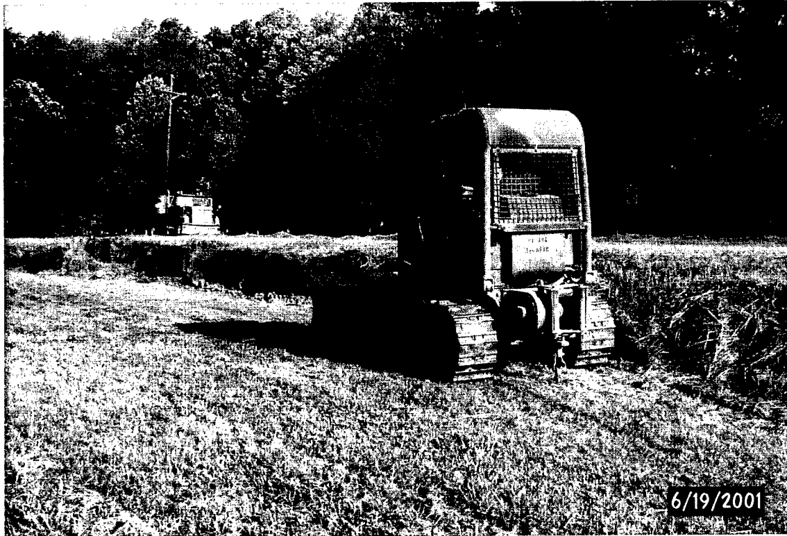
Photo 13. South edge cut at the Susquehana Circle gravel road
