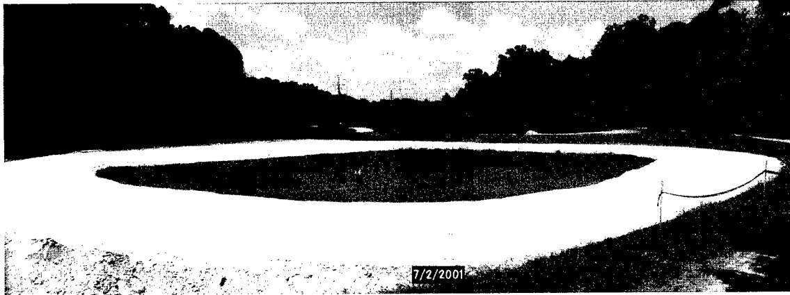
Photo 17. Overall view of the sand layer
