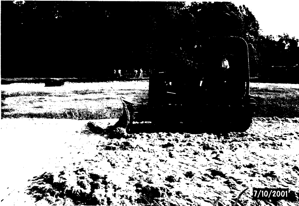
Photo 71. D4 dozer leveling/smoothing the sand-geofiber sections
