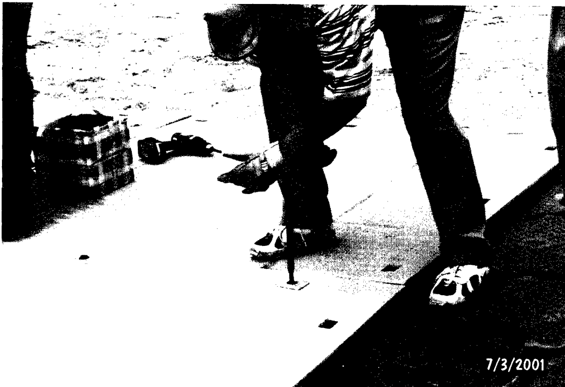
Photo 44. Connector pin pre-tightening using hand tool
