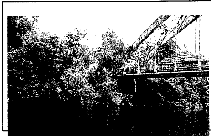
Figure 29. West end of Morey Bridge and bank.
