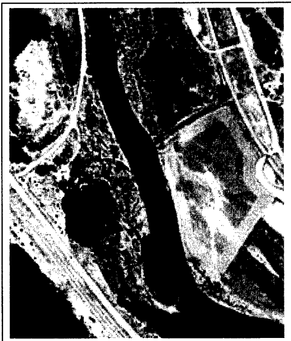
Aerial photo of site 17. The site was initially chosed as a possible AVLB site, but it was too wide.
