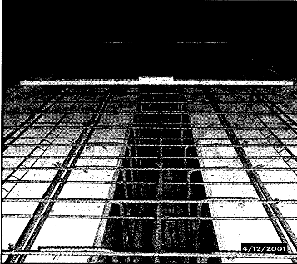
Figure 3.6. Typical Reinforcement Layout
