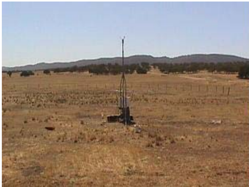
Figure IV.3 Instrumented Portable Meteorological Tower
