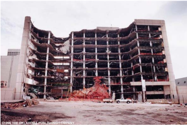
Figure 19 – North View of the Damaged Murrah Building. [23]
