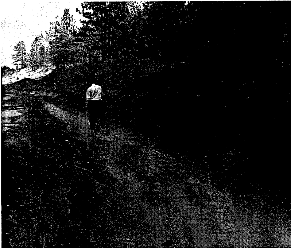
Figure 4. Contaminant migration from washout area at a SAFR berm
