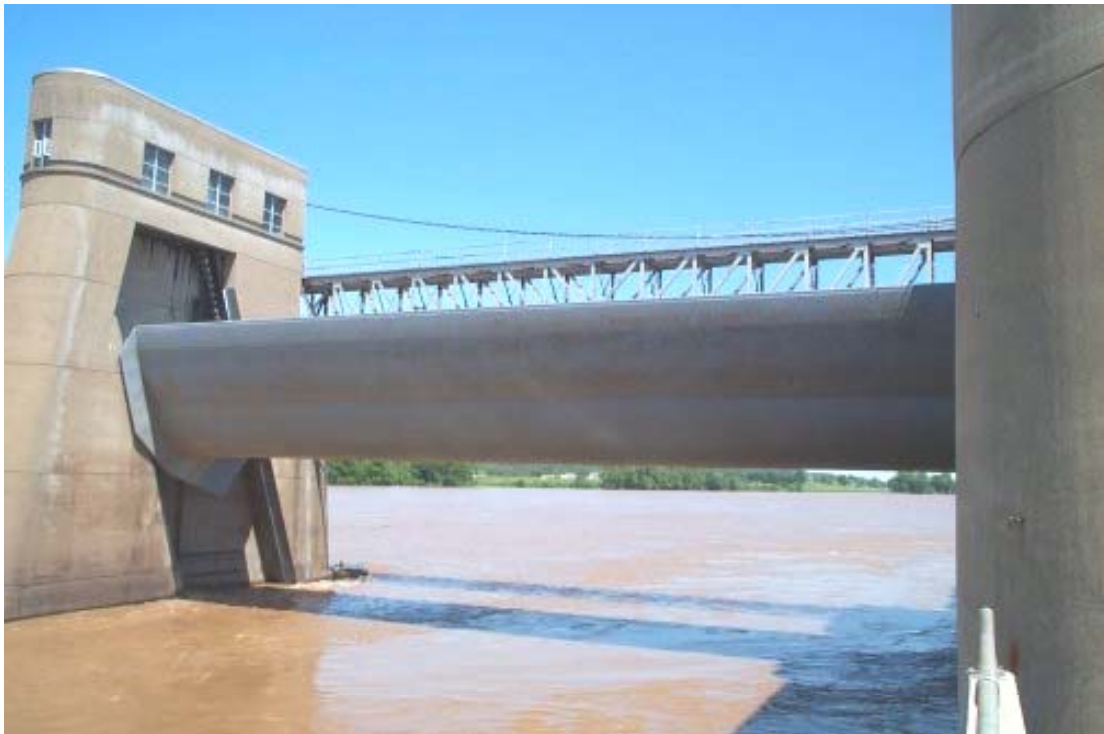
Figure 9. Roller gate installed at R.C. Byrd Dam, Ohio River.
