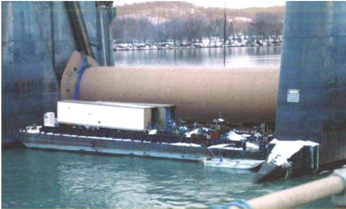
Figure 8. Roller gate being installed at R.C. Byrd Dam on the Ohio River.
