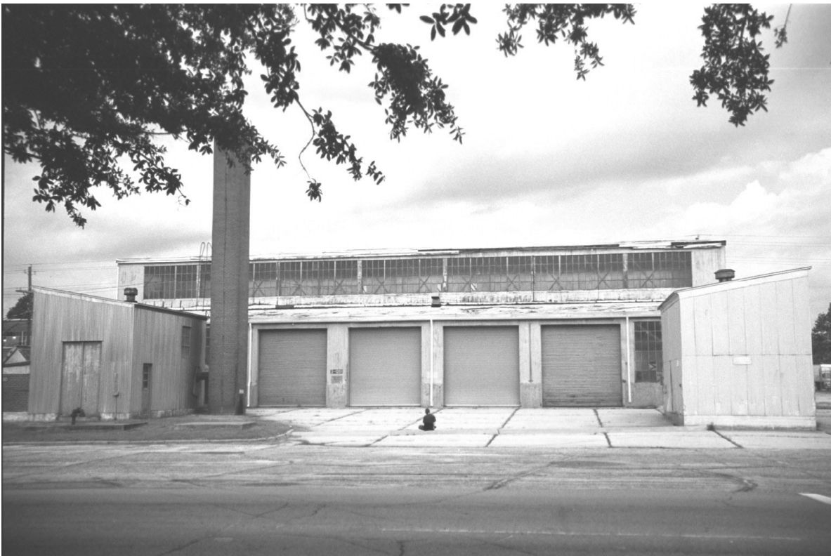
Figure 13: Ordnance Repair Shop with Boiler House on the left and Oil Storage Building on the right (ERDC/CERL).
