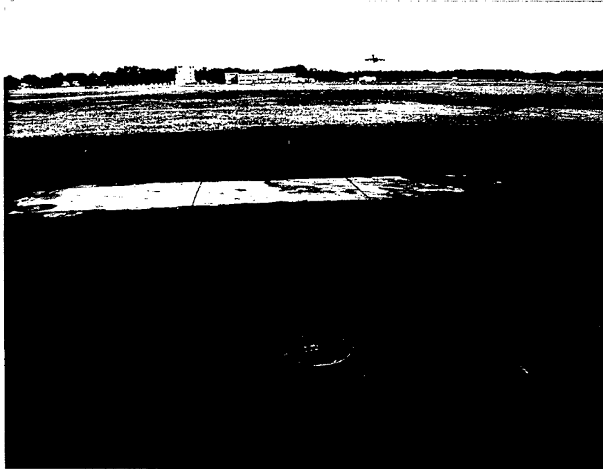
Figure 12. E-Krete and PermaStripe at Norfolk Naval Station. Note the severe hydraulic fluid staining around the concrete island. This area has been used repeatedly for servicing aircraft
