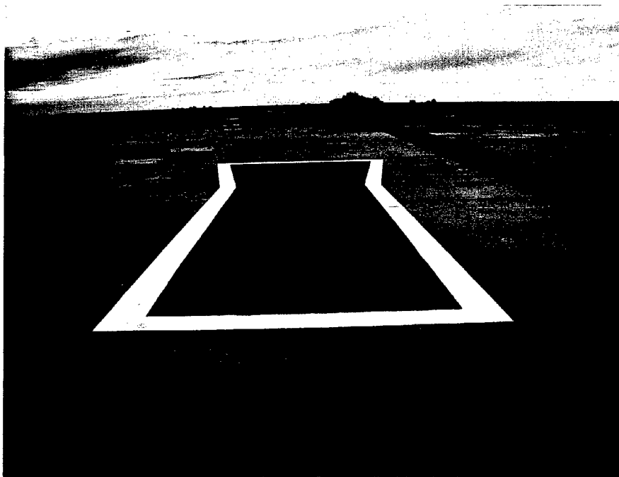
Figure 19. "Red Carpet" area in November 2000. Some fading of the red has occurred and reflective cracks are present, but overall, this section is in excellent condition
