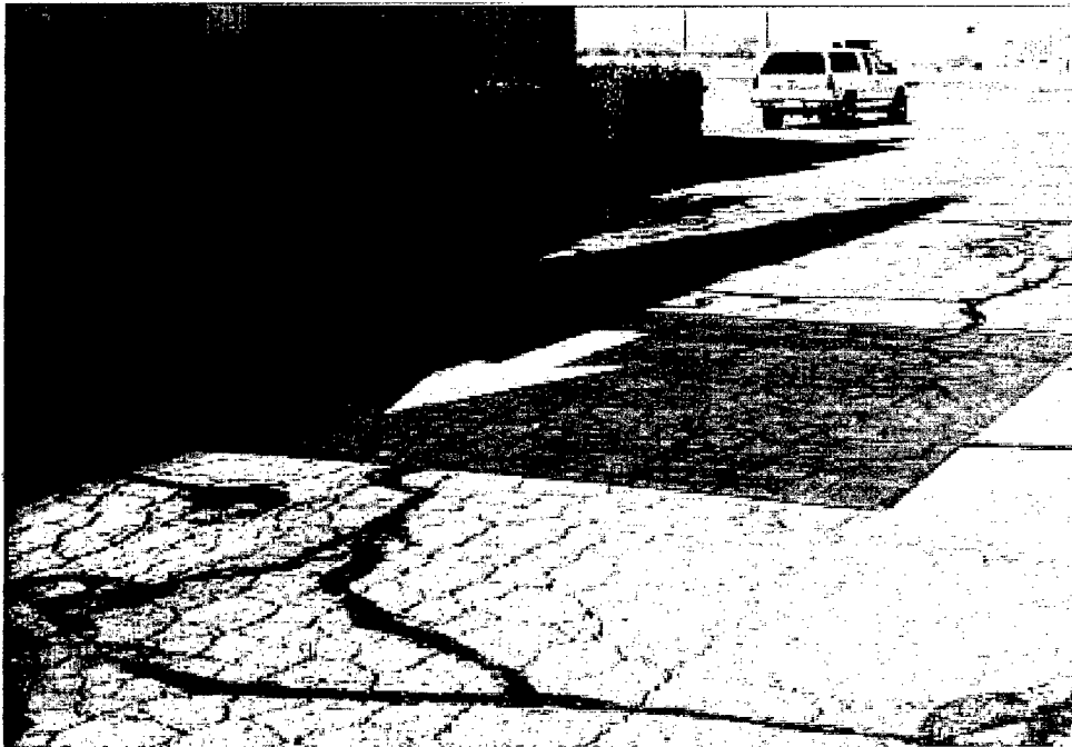
Figure 14. E-Krete and PermaStripe at Edwards AFB. Note the severely cracked asphalt surface upon which the E-Krete was placed. Although many of the cracks have reflected back up through the E-Krete, it is in much better condition than the asphalt with virtually no raveling, unlike the surrounding pavement
