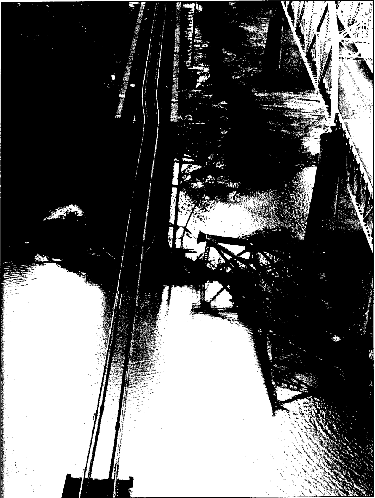
Flooded railroad bridge over the Missouri River near Glasgow, Mo.
