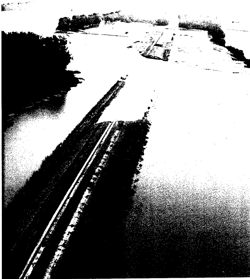
Federal Levee L246 at RM 241 on the Missouri River.
