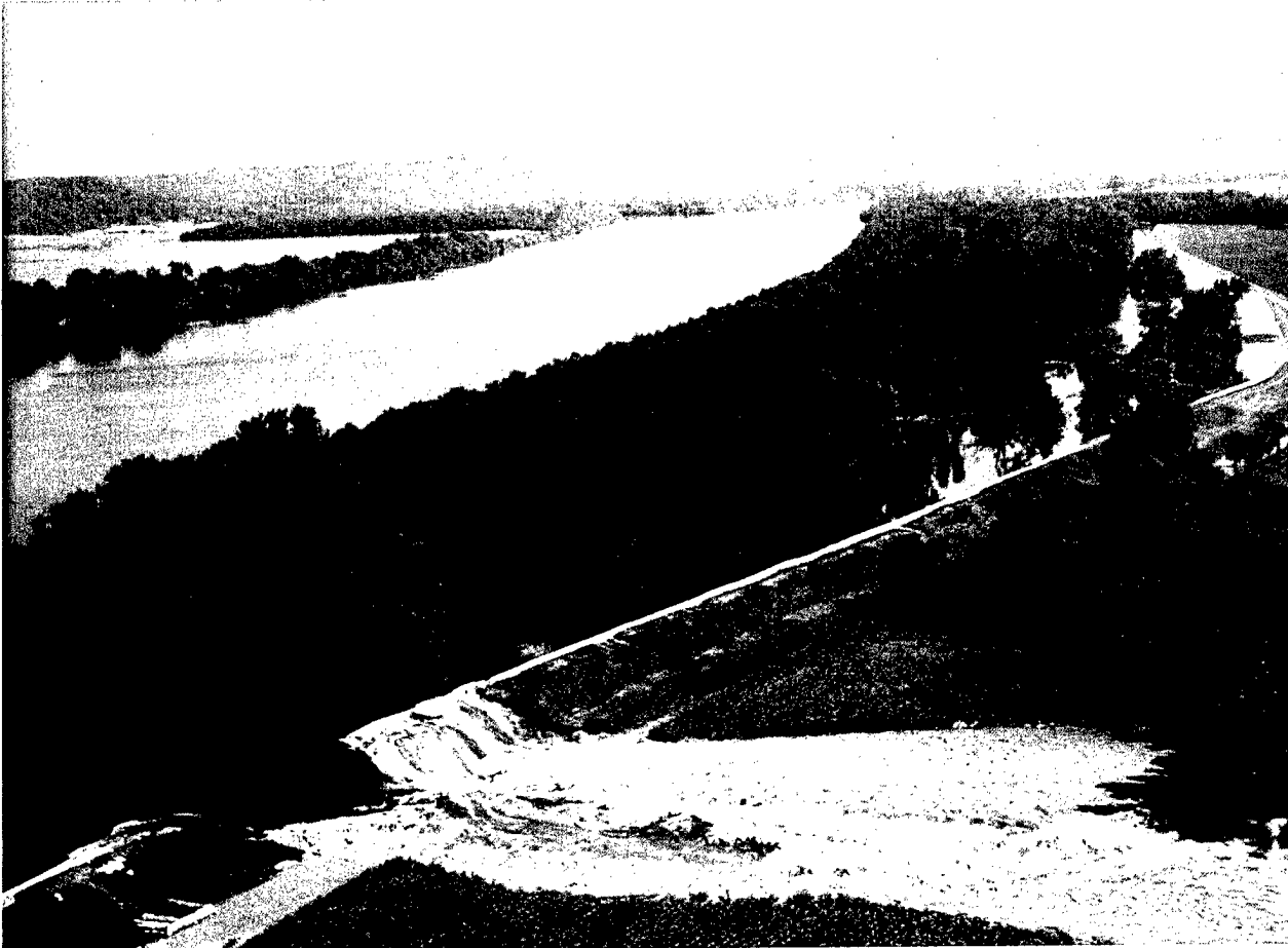
Nutwood Levee break on the Illinois River.
