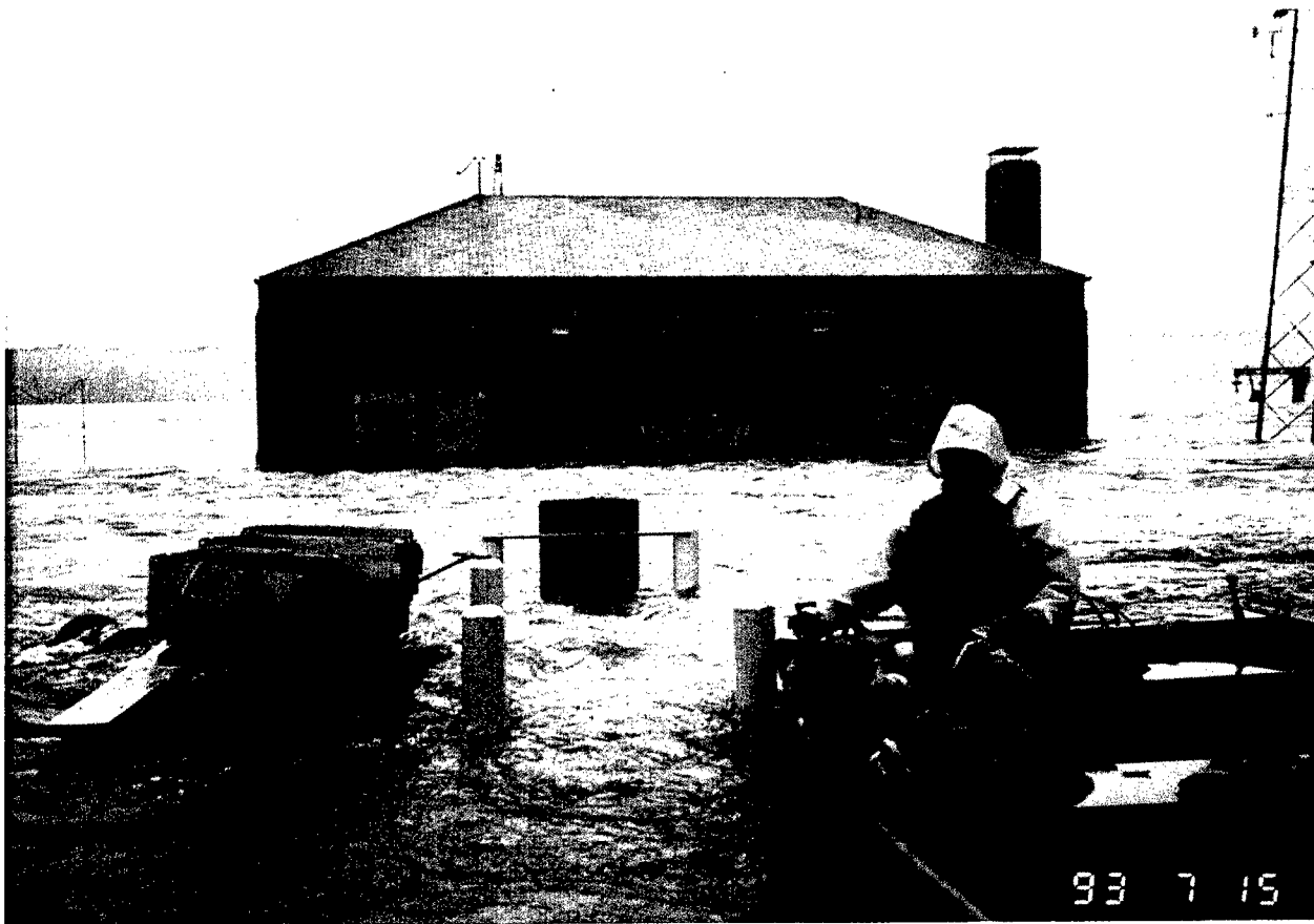
Flooded control house at Lock and Dam 21, Quincy, Ill.
