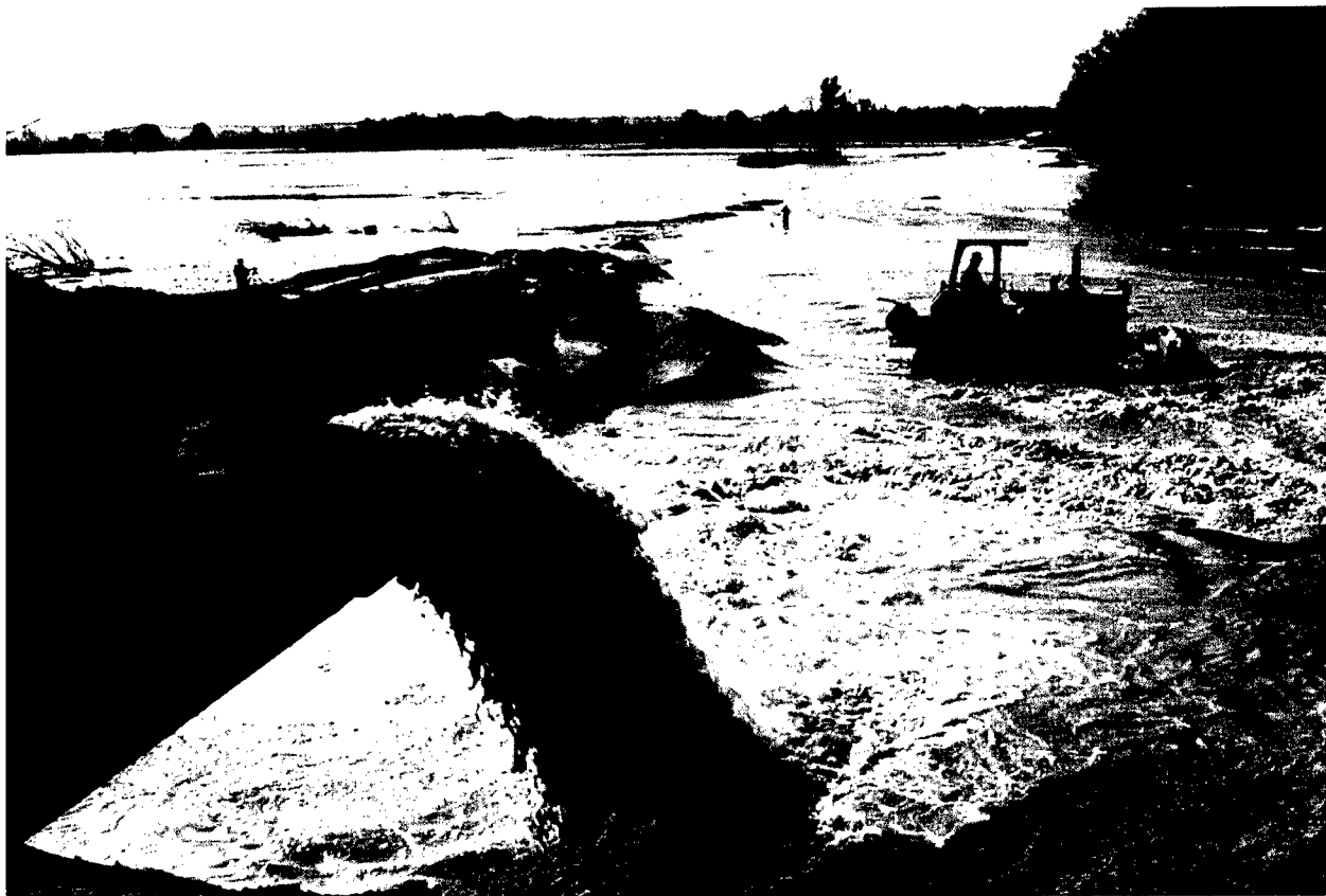
Hydraulic dredges repairing the damaged Sny levee.
