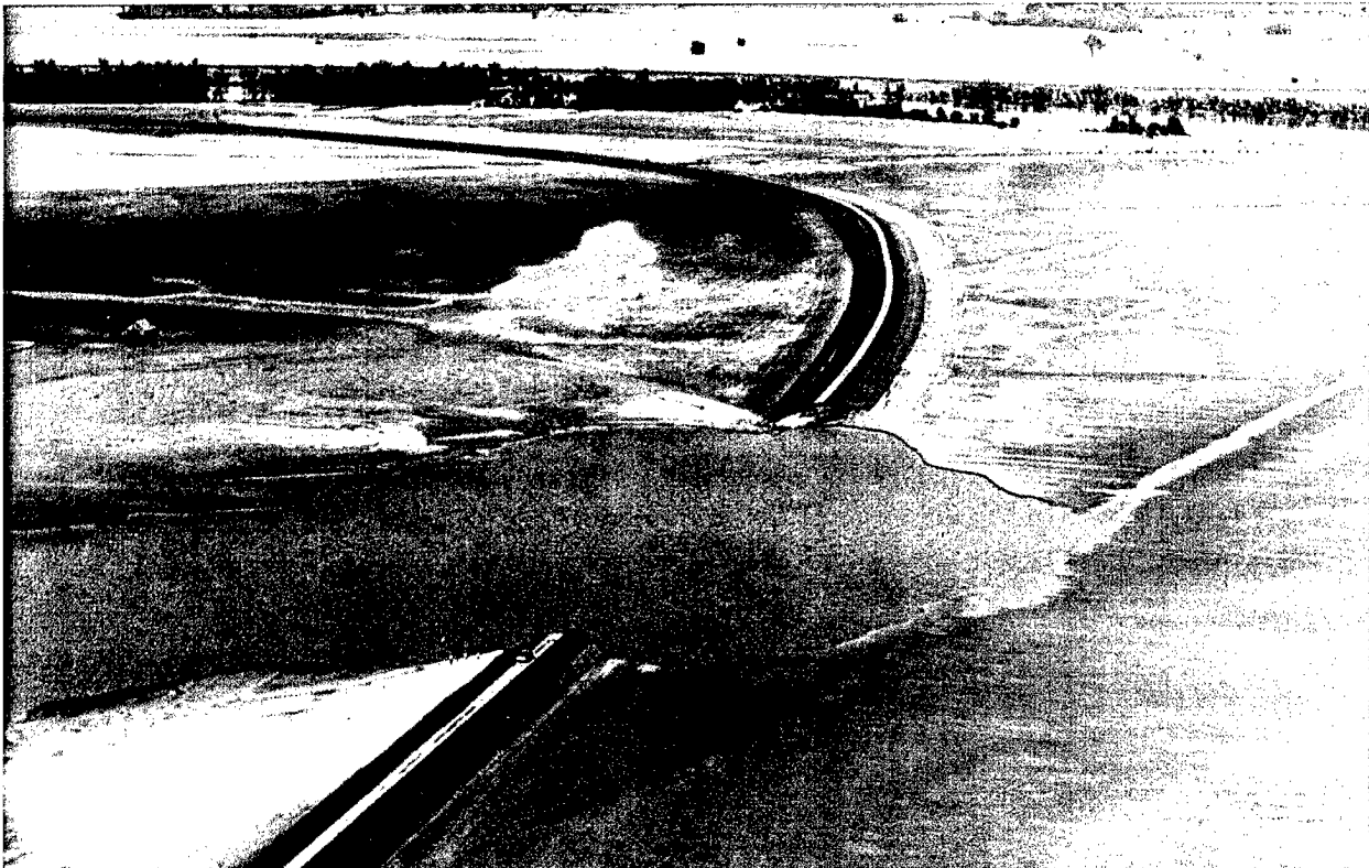
Levee breach at L470-460 near Elwood, Kan.
