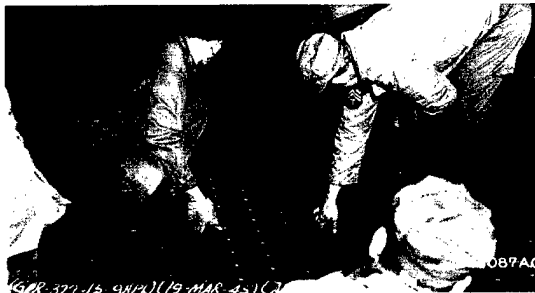
(a) Pierced Steel Planking (PSP) being installed at night by men of the IX Engineer Command at an Air Force Base in Germany (circa 1945).
