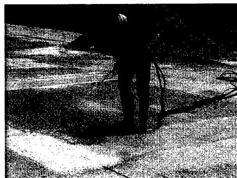
(e) Spraying to 6-mm ( \frac{1}{4} ") thickness
