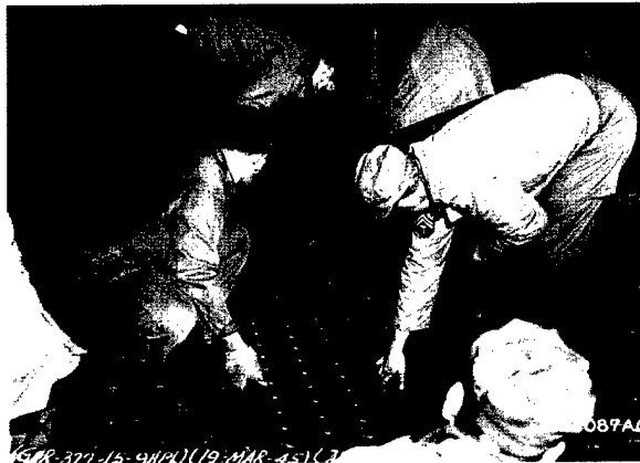
Figure 1. Pierced Steel Planking (PSP) being installed at night by men of the IX Engineer Command at an Air Force Base in Germany (circa 1945).
