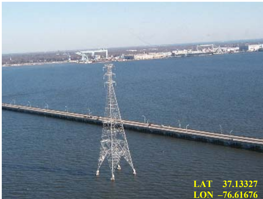
FIGURE 4: JAMES RIVER BRIDGE (WIRE SET #1) 6 LARGE WIRES AND 2 SMALLER GUIDE WIRES EASILY DETECTED VISUALLY WITH NO BACKGROUND
