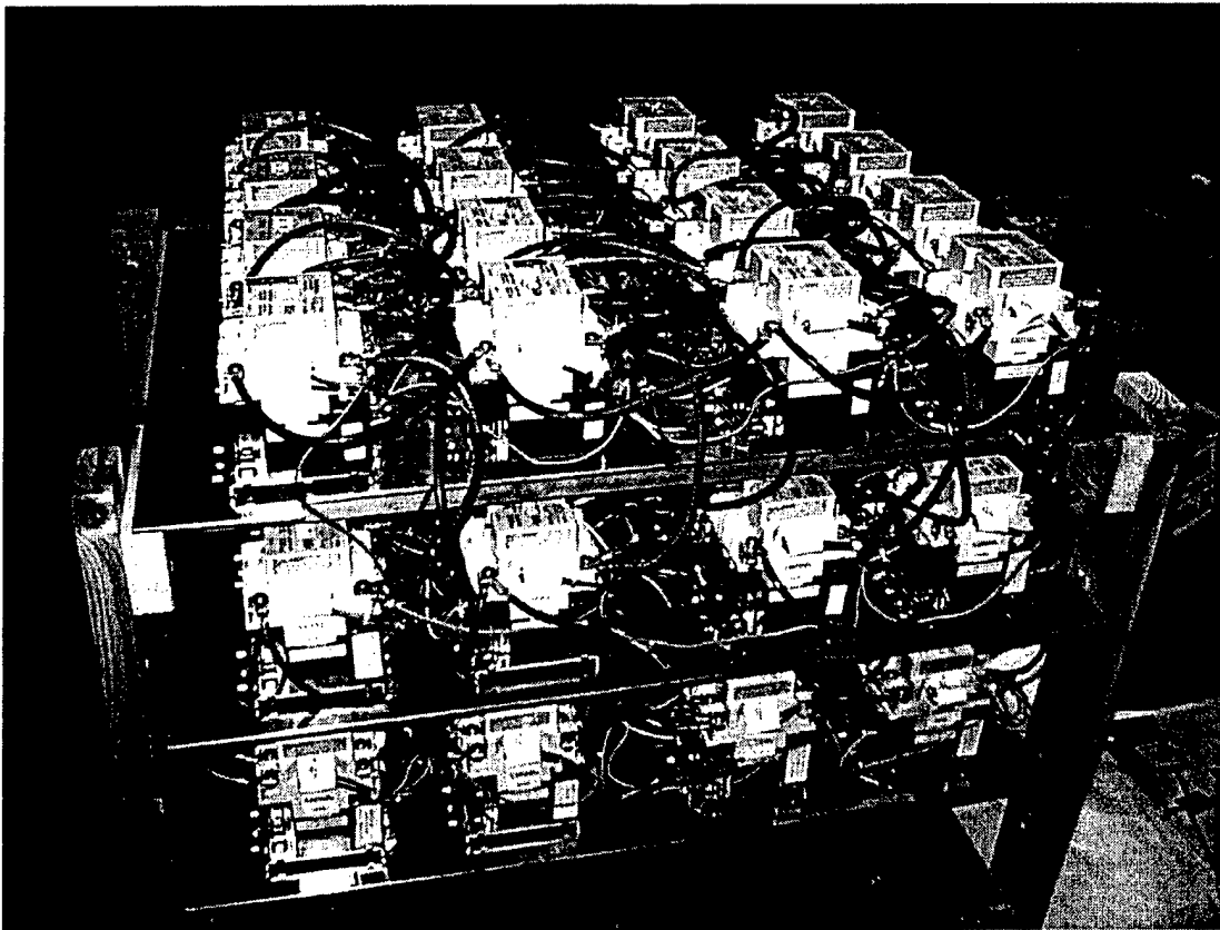
Figure 3. New Electrical Contactor Configuration for NetSim
