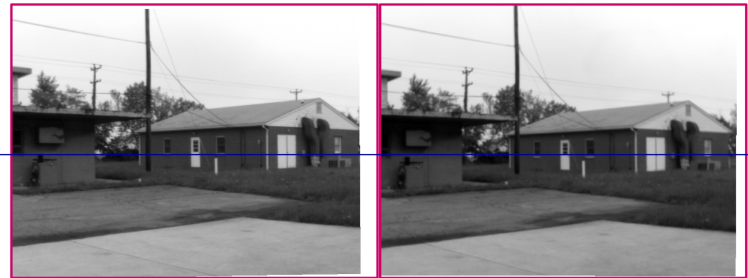
Figure 29. Rectified image pair for the building image pair with calibration image set 3 parameters.
