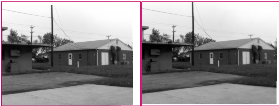
Figure 31. Rectified image pair for the building image pair with calibration image set 5 parameters.
