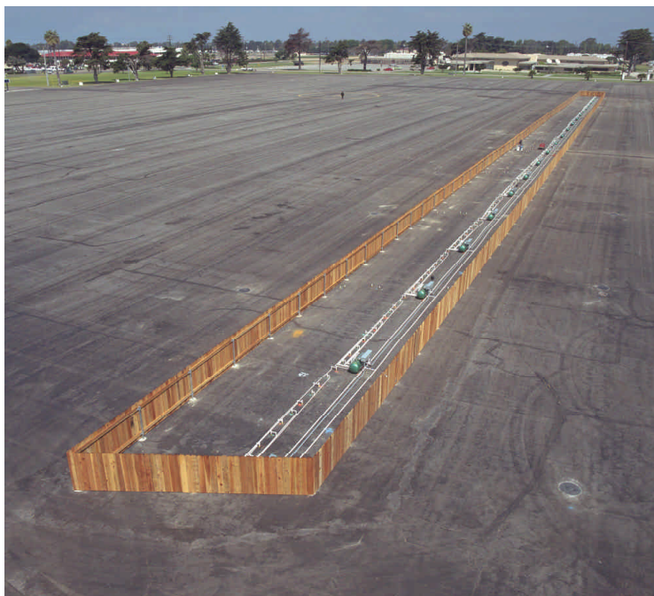
Figure 1. Bio-barrier located at NBVC, Port Hueneme, California.
