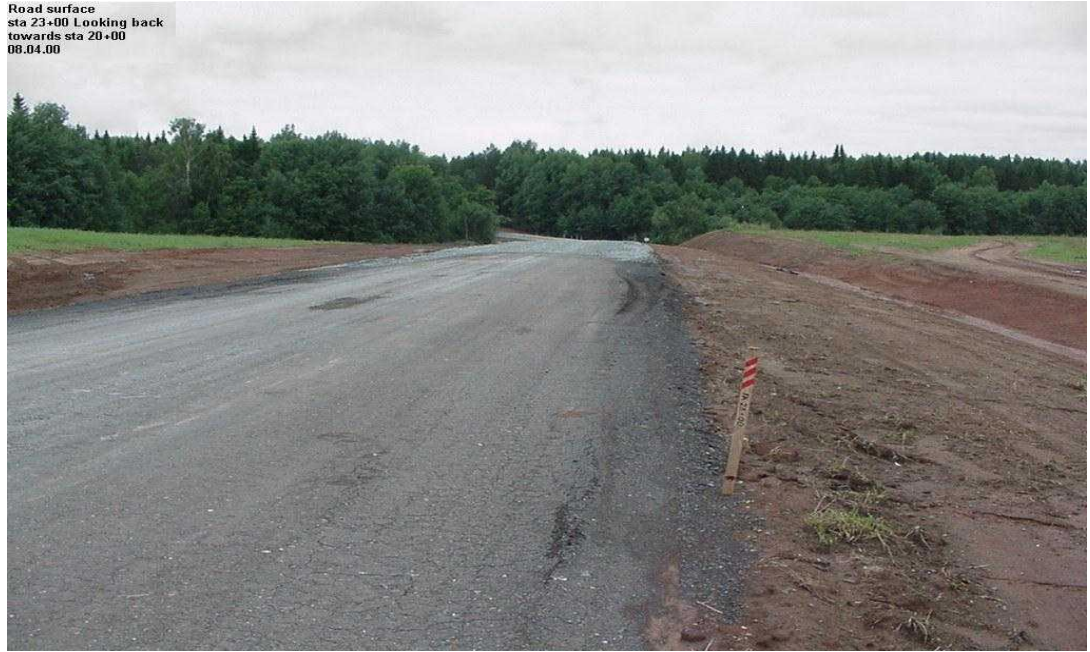
Figure C-4. Portion of the 4-kilometer gravel access road
