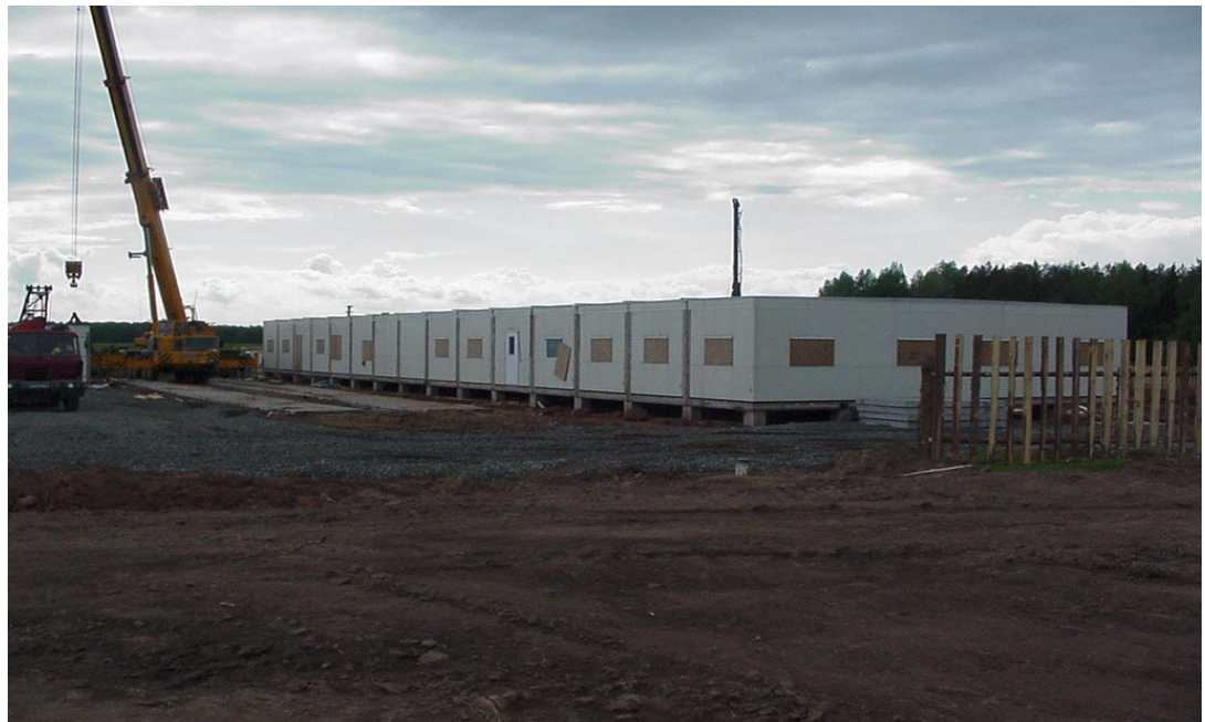
Figure C-1. Administrative building (Building 5) during construction
