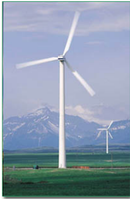
Figure 2. A Horizontal-axis Three-bladed Turbine (Vision Quest Windelectric, 2003)
