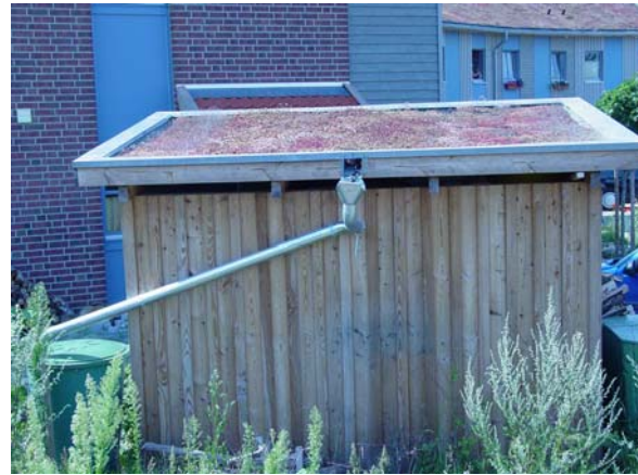
Figure 4.24 Refuse Shelter. The water retention benefits and aesthetics of vegetated roofing make it worthwhile for Germans to install vegetation on small refuse sheds.
