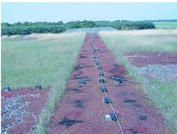
Figure 4.19 Building 3. The Building 3 roof has varying conditions such as exposed gravel, no soil, and multiple soil depths.
