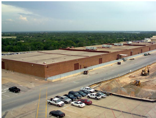
Figure 4.1 Building 15 at AFP 4 in Ft. Worth, TX. Building 15 has over 100,000 ft 2 of roof. (Rowls, 2003)
