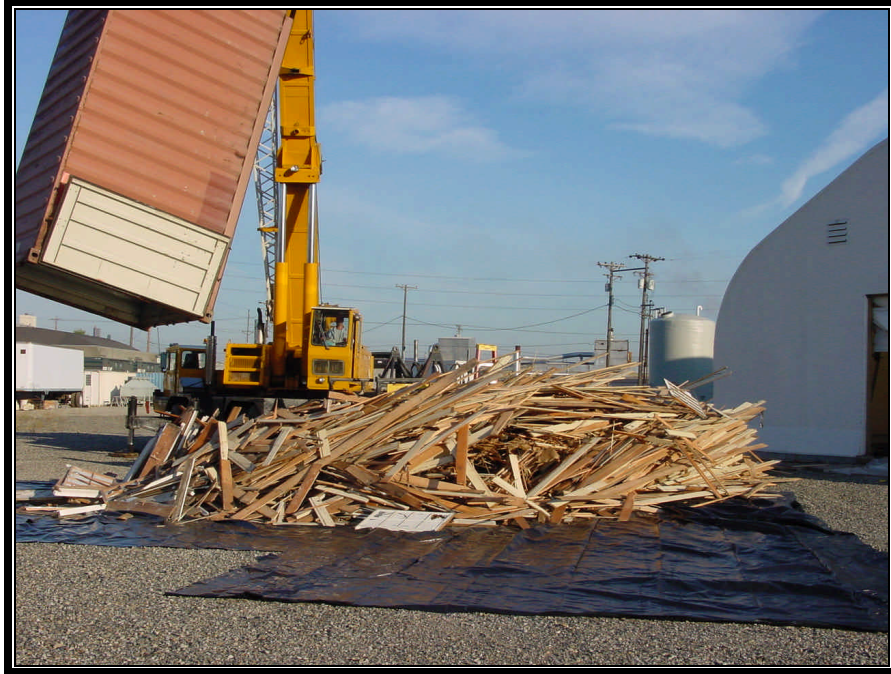
Figure 7. Ft. Ord Debris Unloaded from Shipping Container
