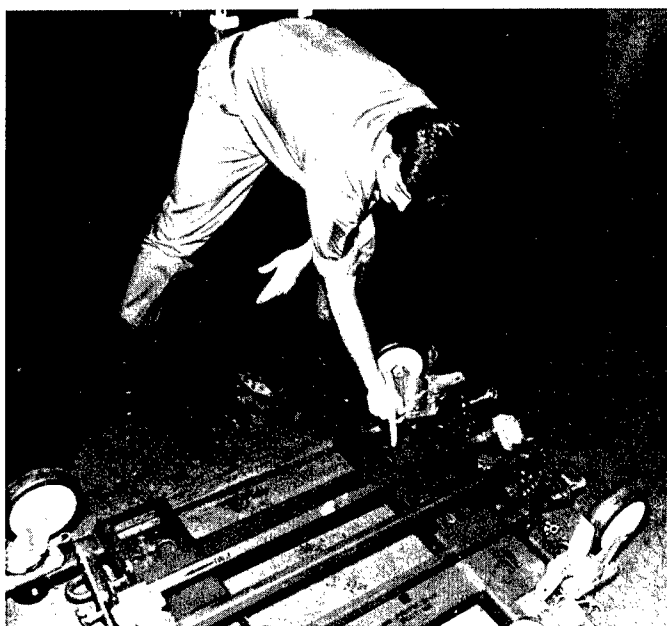
"Only use the right side." Fit, Form and Function testing for support equipment actually works. This AGM-130 missile cradle assembly had to be modified to ensure accessibility from both sides.
