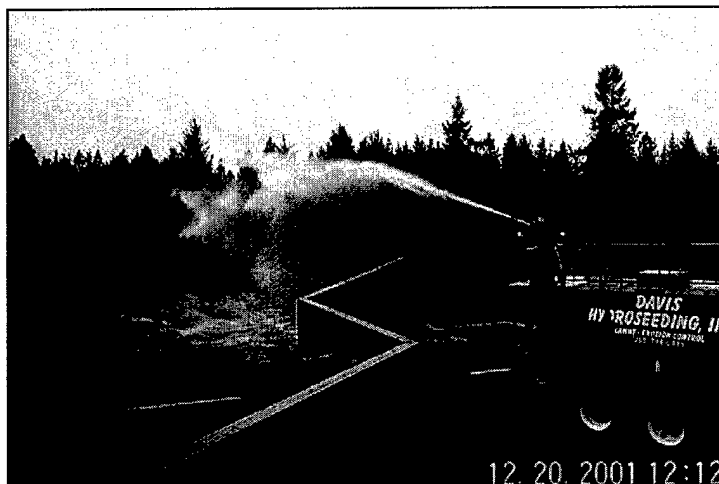
Figure 5. Lime application using a hydro-seed spreading cannon.
