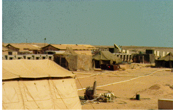
Figure 26. Above-Ground Water Distribution Hoses.
