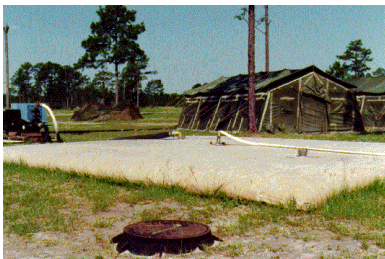
Figure 25. Water Storage Bladder.
