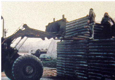
Figure 12. Aircraft Revetment Erection.
