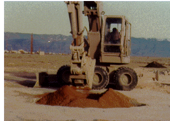
Figure 4. Pavement Repairs. Equipment).
