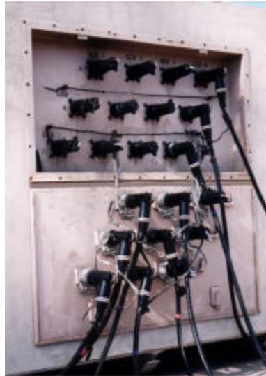
Figure 48. Primary Cable PDC Line Side Connection.
