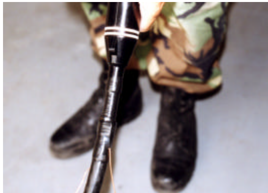
Figure A4.16. Wrap the End of the Elbow for Protection.
