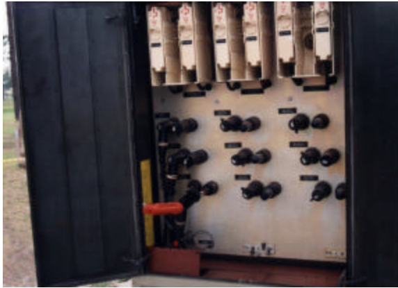
Figure 51. Remove the Center Pole of SDC Fusible Disconnect Switches.
