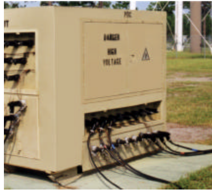
Figure 54. Arc Strangler Switches Removed from Unused PDC Feeders.
