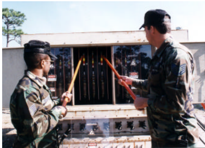
Figure 60. Proper Set-up for Disconnecting the Arc Strangler Switches.
