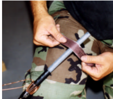
Figure A4.4. Sand and Clean the Insulation to Remove Marring.
