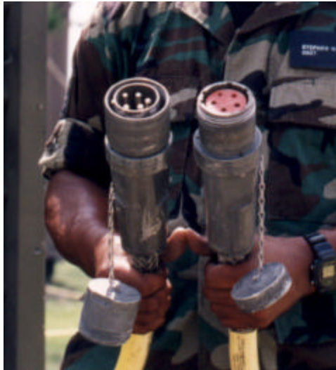
Figure 11. Cannon Plug Connections on Low Voltage Cable.
