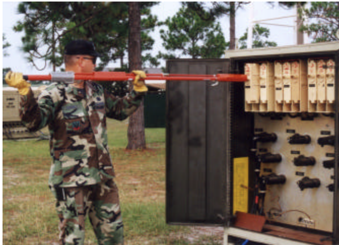
Figure 62. EFD Center Pole Disconnect with a Switch Stick.
