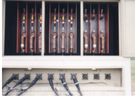
Figure 54. Arc Strangler Switches Removed from Unused PDC Feeders.
