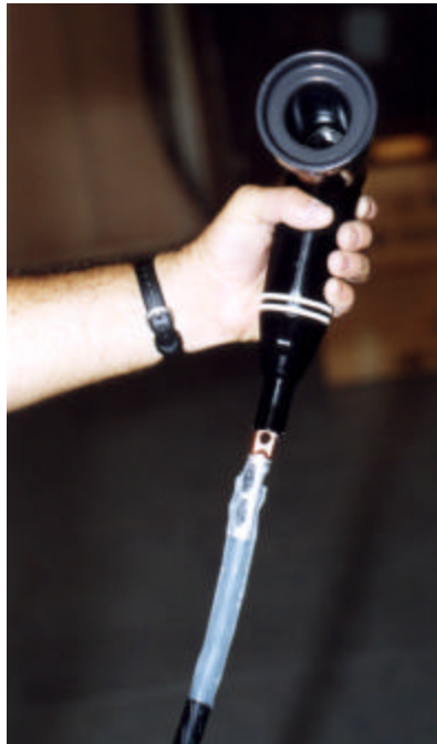
Figure A4.11. Apply Small Amount of Silicon Grease to Exposed Cable before Assembly.
