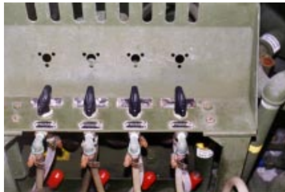
Figure 37. Chemical Feed Run/Prime Values in PRIME Position.
