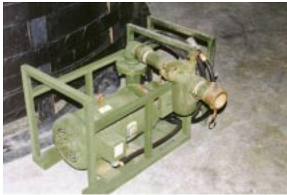
Figure 23. Backwash Pump Assembly.
