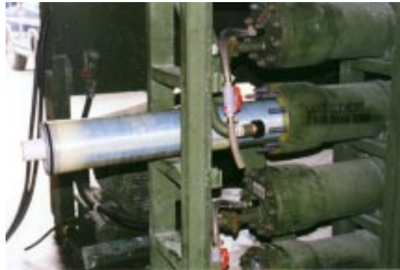
Figure 51. Insertion of R.O. Element into Pressure Tube.
