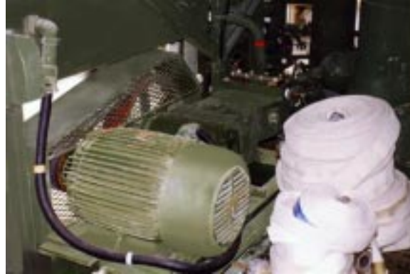
Figure 7. Reverse Osmosis Pump Assembly.
