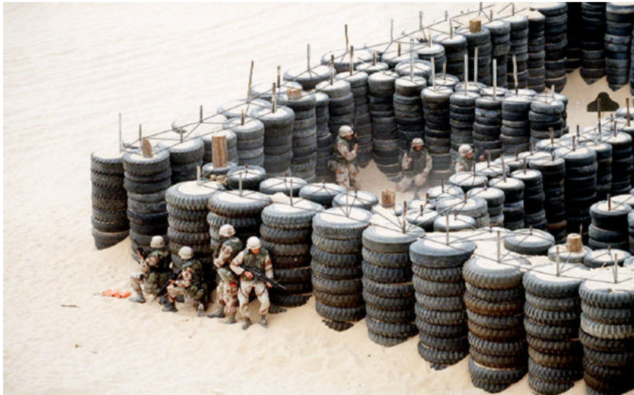
Figure 24. Tire Revetment Walls.
