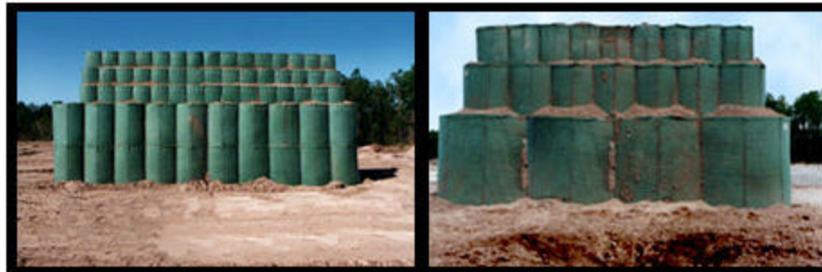
Figure 36. Wire Frame, Fabric-Lined Container/Concertainer Revetment.
