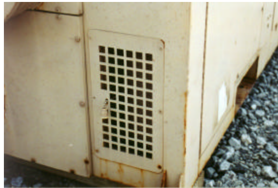
Figure 33. Manually-Operated Damper.
