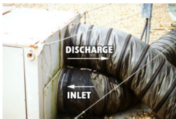
Figure 30. Flexible Duct Connection.
