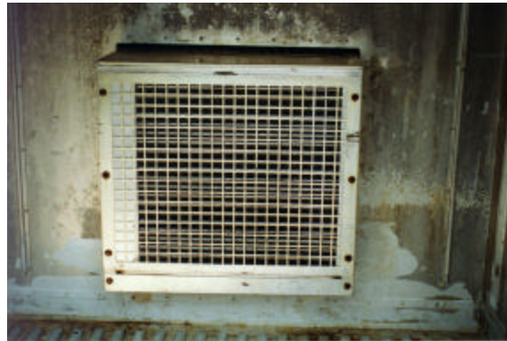
Figure 41. Evaporator Coil.
