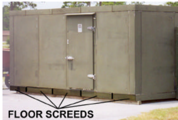
Figure 51. Floor Screed Section.
