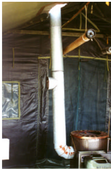
Figure 26. Stove Pipe Assembly.
