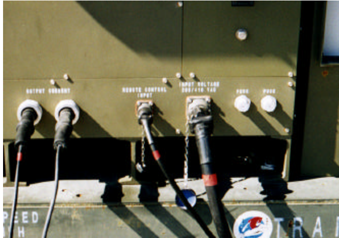
Figure 35. P11/J11 Connection on Generator.
