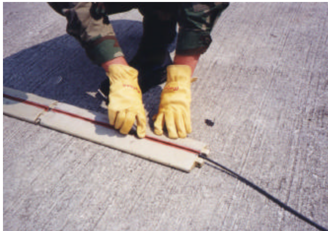
Figure 24. Laying Cable in Cable Protection Strips.
