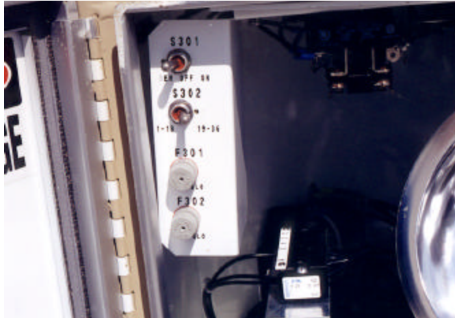
Figure 16. Strobe Master with Series Circuit Adapter.
