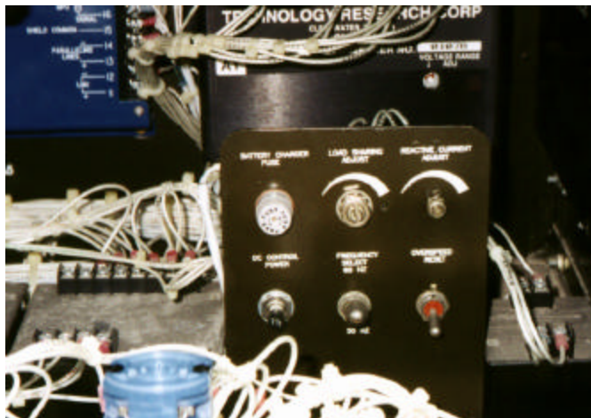
Figure 39. Control Bracket Behind Generator Control Panel.
