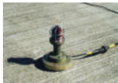
Fixture uses split red / green glass lens, 120W lamp, and 100W IL
