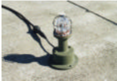
Fixture uses clear glass lens, 45W lamp, and 45W IL
