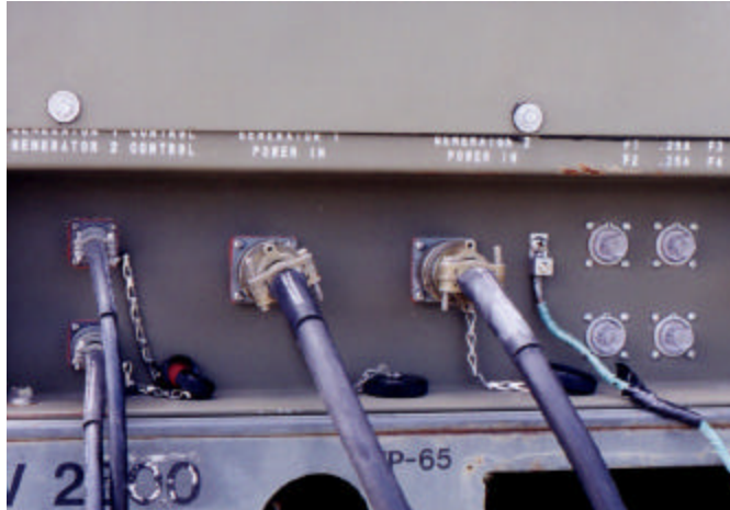
Figure 33. Cable Connections from Control Panel to Regulator.
