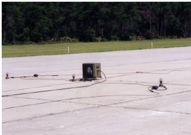
Figure 18. Approach Cross Bar.
