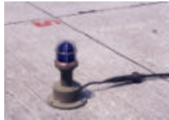
Uses blue glass lens, 30W lamp, and 45W IL
