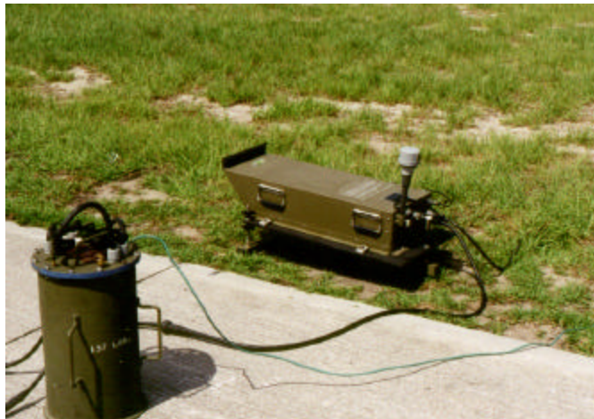
Figure 20. Inboard PAPI and Series Circuit Adapter.
