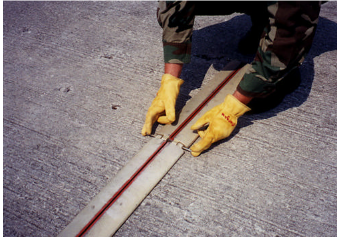
Figure 24. Laying Cable in Cable Protection Strips.
