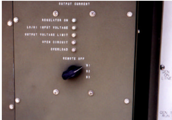
Figure 41. Backup Control Panel and Regulator Panel.
