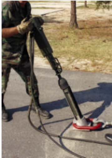
Figure 27. Driving a Stake with Hydraulic Breaker.
