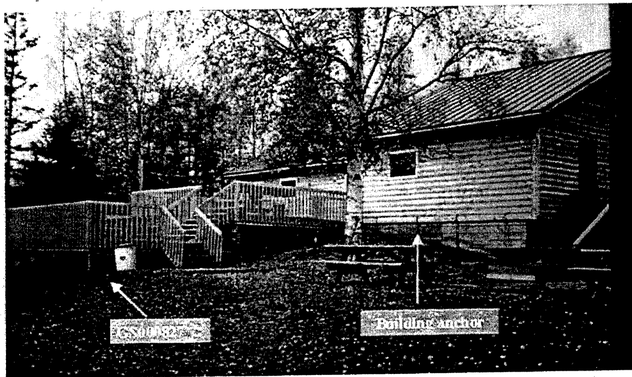
Figure C-1: Back of MAC Chalet. Photograph taken while standing on 702WL04.
