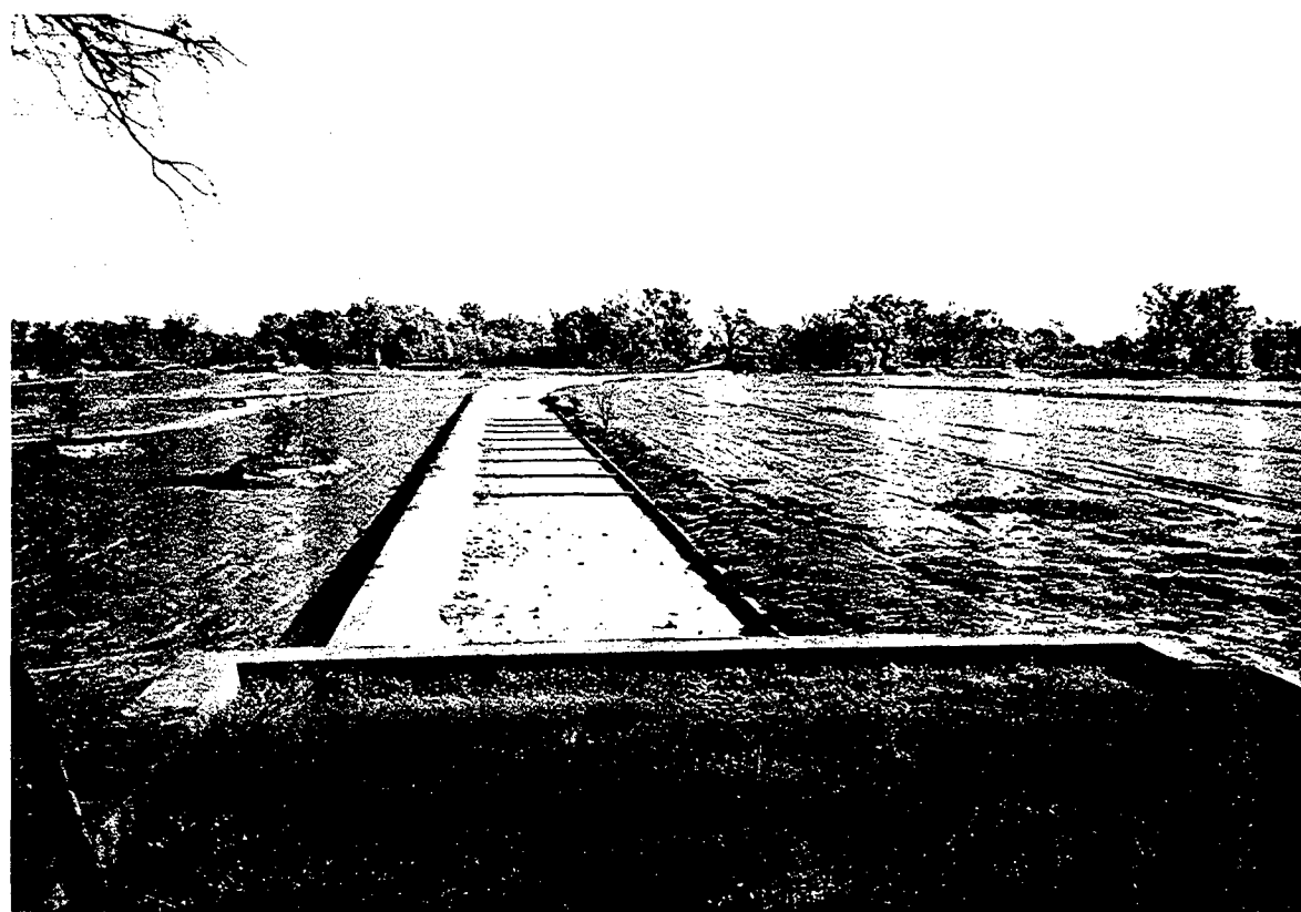
ACCUMULATED DEBRIS AND SEDIMENT IN VICINITY OF FREMONT WEIR WAS REMOVED BY STATE AFTER FEBRUARY 1986 FLOOD.
